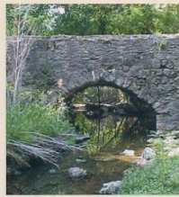
Aqueduct carrying Espada acequia over San Pedras Creek
