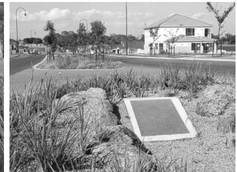
When the discharge capacity of the system is exceeded stormwater is conveyed as open channel flow. Culverts are used to convey these flows under vehicle turnings.
