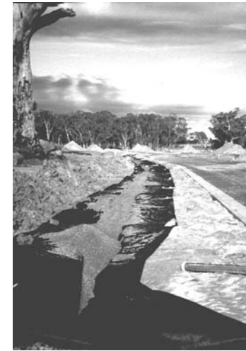
Backfilling of the trench with gravel screenings 4-7mm in diameter.
