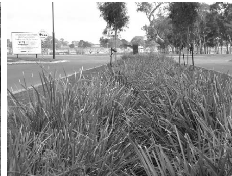
Thick tussock grass provides further treatment to road runoff prior to entering the gravel trench.
