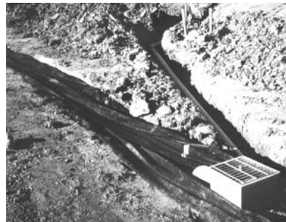
Roof runoff is conveyed to driveway inlet pits, which are also used to discharge surface flows that exceed the infiltration capacity of the grass swale.
