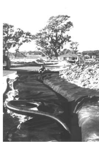
Laying of the geotextile fabric and 150mm diameter perforated pipe.
