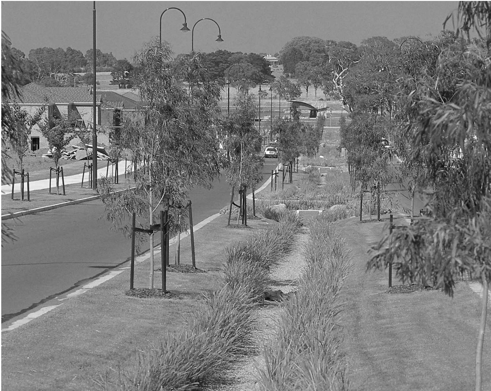
Bio-filtration system along Lynbrook Boulevard at Lynbrook Estate, Victoria
