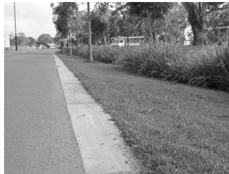
No kerb and gutter system promotes an even distribution of flow from the road surface onto the grass filter strip for pre-treatment.
