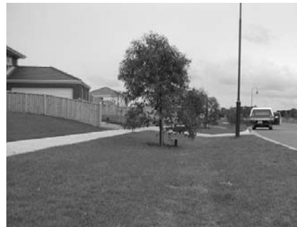
The grassed swale forms the nature strip. Road runoff is diverted onto the swale from the kerb and gutter system using kerb inlet chutes located on the downstream side of each driveway cross over.
