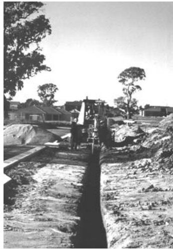
Excavation of the trench component of the bio-filtration system.
