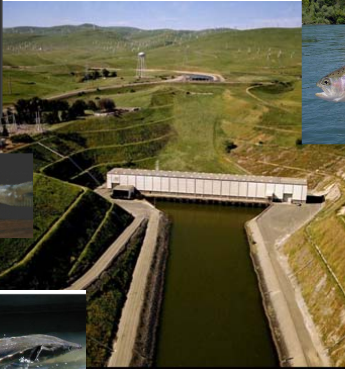
Banks Pumping Plant State Water Project
