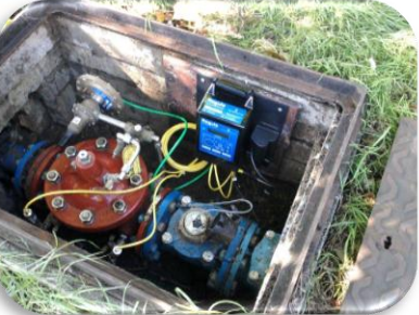
DISTRICT METER CHAMBER INSTALLATION
