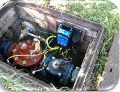
DISTRICT METER CHAMBER INSTALLATION
