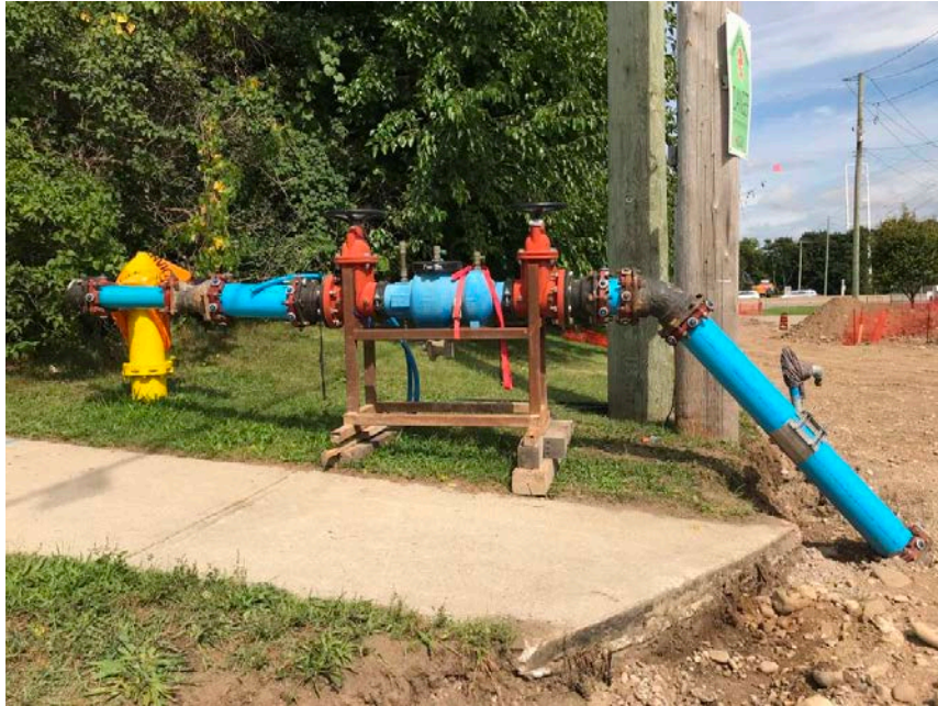
Figure A-1: Temporary connection from a hydrant with Backflow Prevention using a CSA-certified reduced pressure principle backflow preventer.
