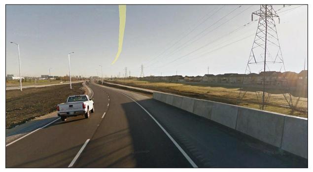
Figure 10: High voltage tower out of clear zone, but extending F-shape barrier from bridge provides increased protection as well as other benefits.
