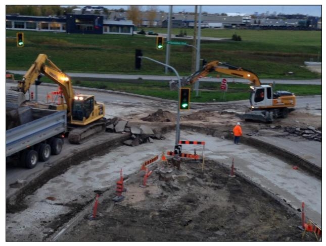
Figure 15: Removing the temporary granular and asphalt roadway surface that provided needed superelevation for the Southbound to Eastbound curve.
