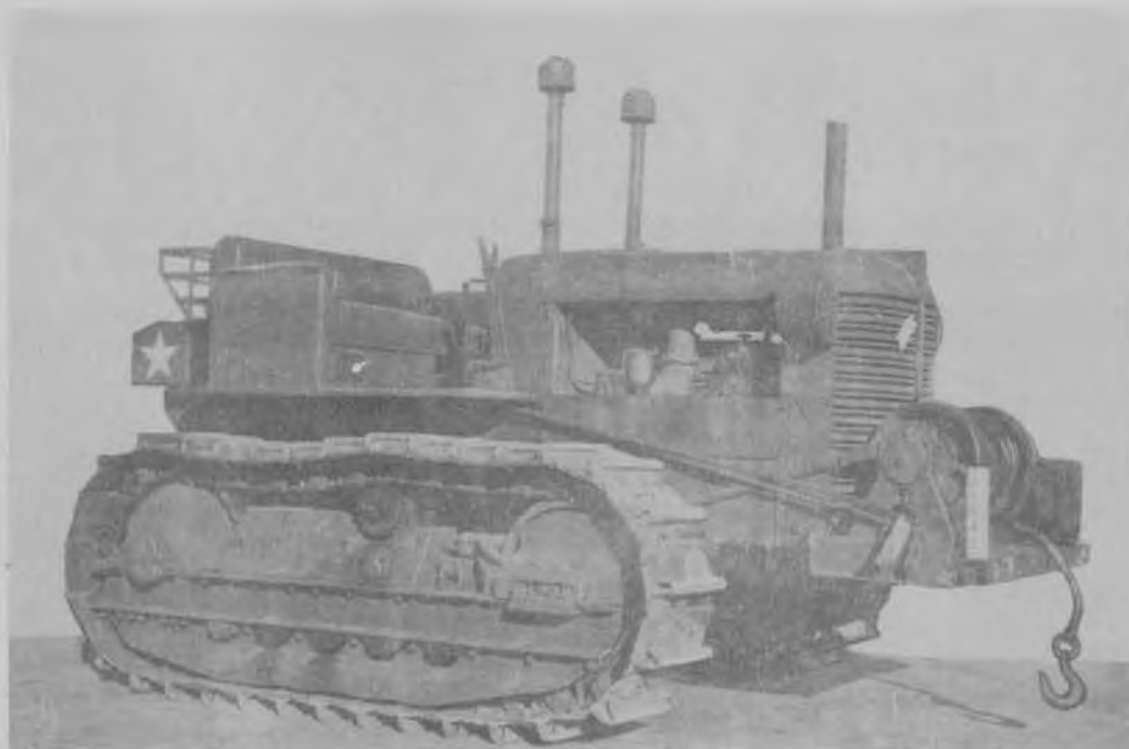
TRACTOR, TD-14, WITH FRONT MOUNTED WINCH
