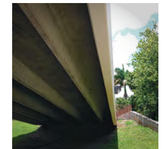
PARKING GARAGE RAMP NEAR COLUMBIA VILLAGE
