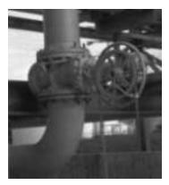
The chainwheels have an extra deep channel in which the chain runs to assure that the chain will not climb off the track.
