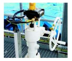
General Twin Seal can be fitted with switches or sensors to provide Open/Closed position indication of the valve.
