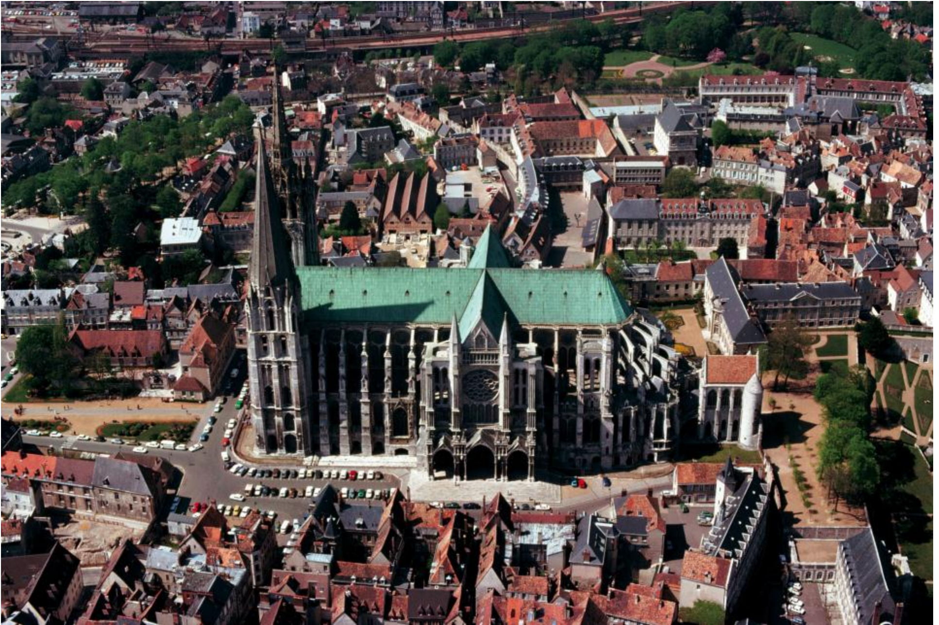
Aerial view of Chartres Cathedral (looking north), Chartres, France, as rebuilt after 1194
