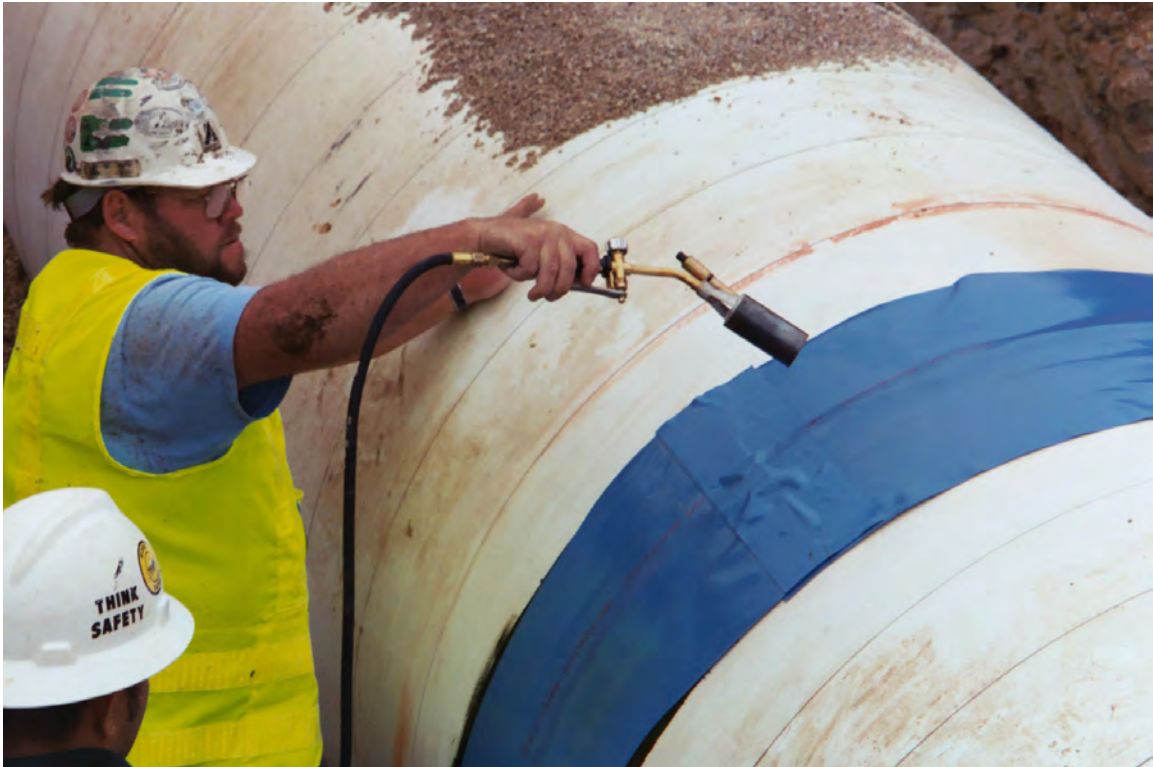
Applying a heat-shrinkable coating.
