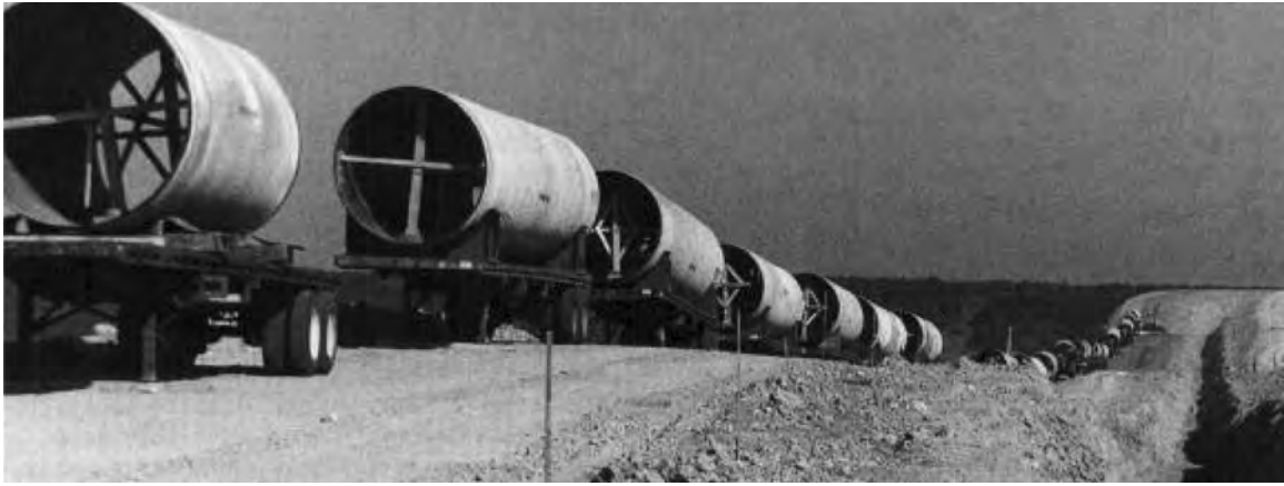
San Diego, Calif. 96-inch I.D. Pipe
