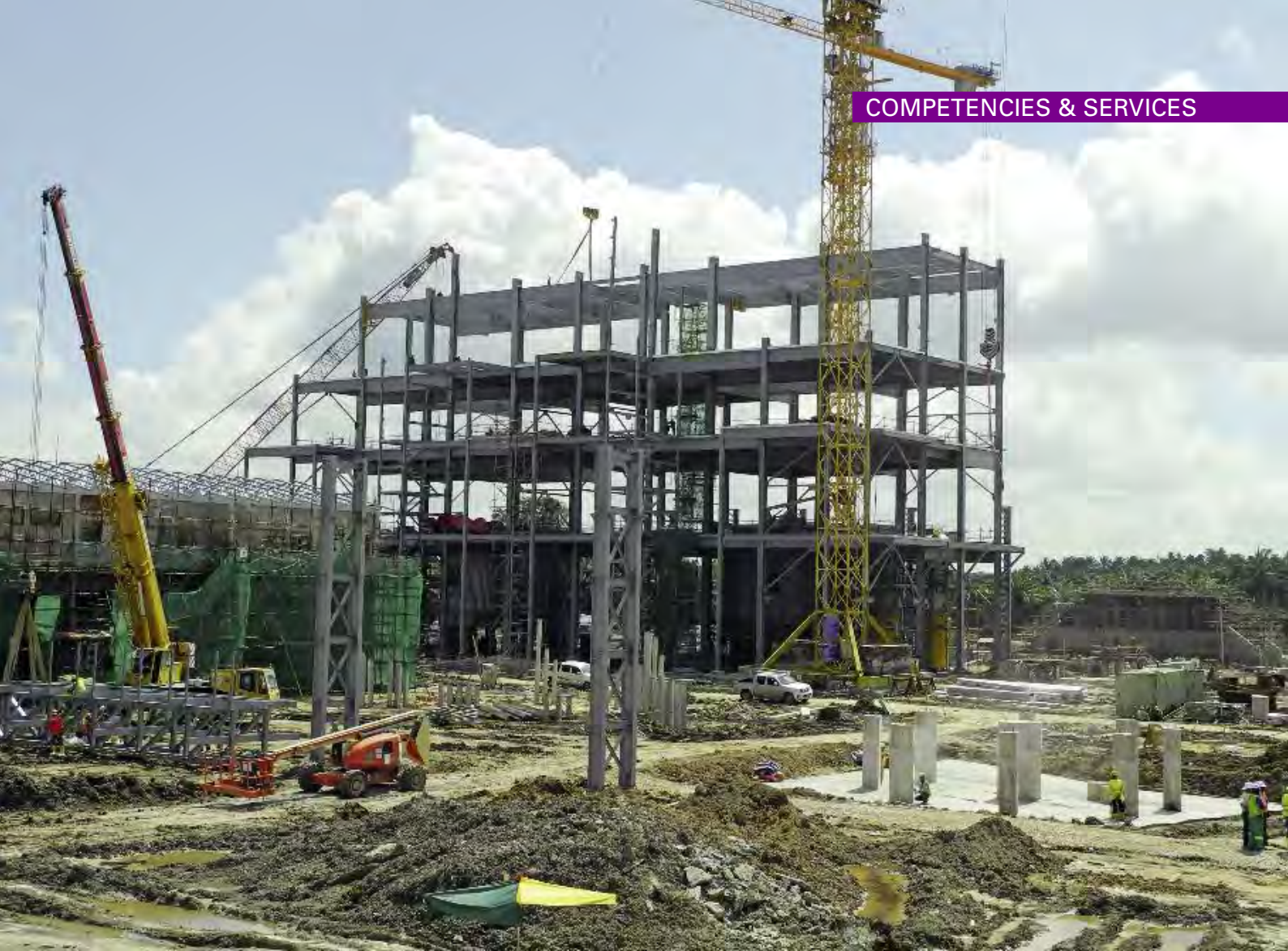
FeMn plant during construction.
