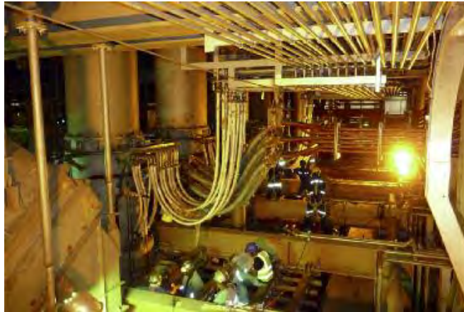
Installation of furnace for FQM.
