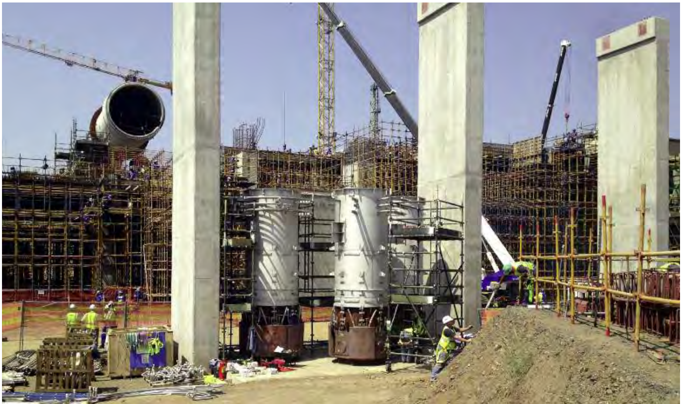
Xstrata Lion 2 project during construction.
