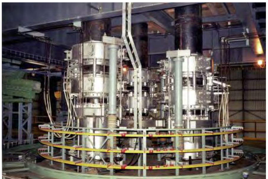
Roof section of copper slag cleaning furnace.
