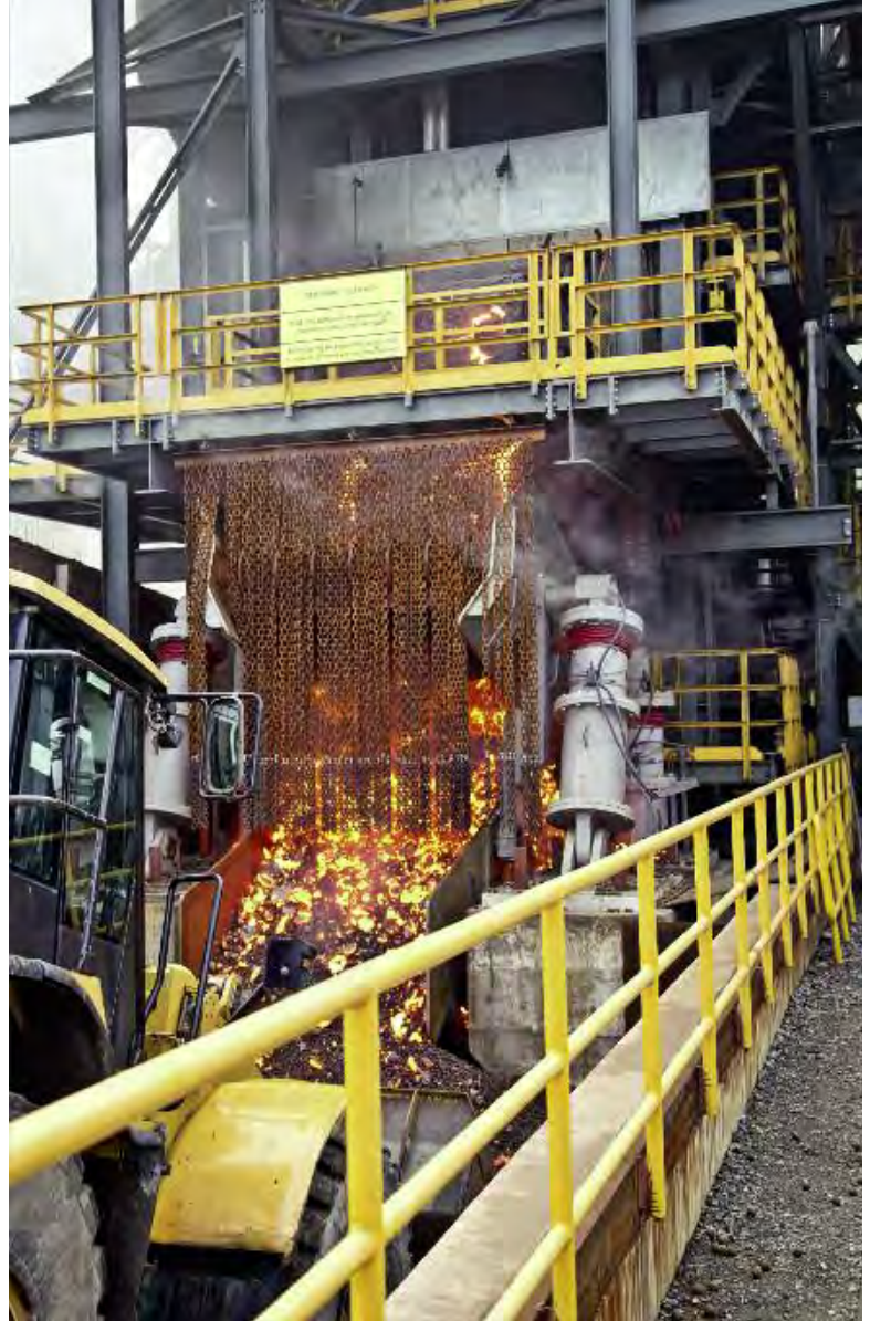
Dry slag granulation (Dillingen) Pilot plant startup.
