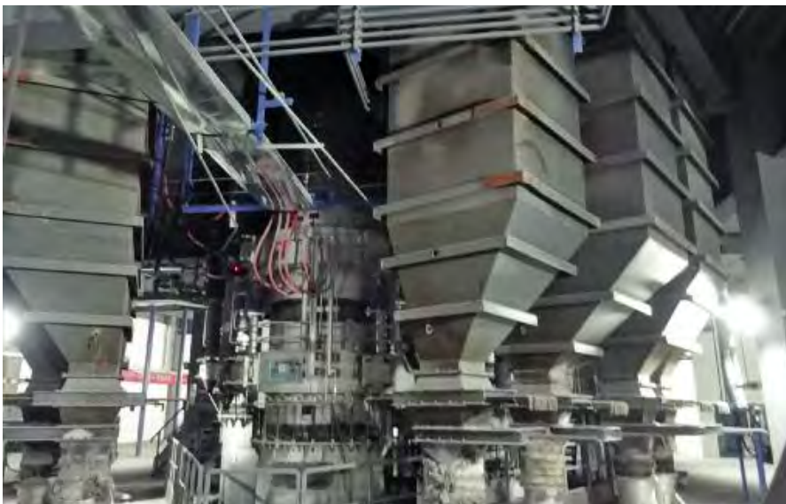
Installation of electrode column.
