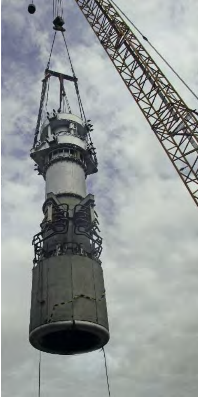
Electrode column during installation at PT Antam.
