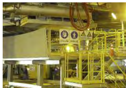
Mudgun and drilling machine (TMT).
