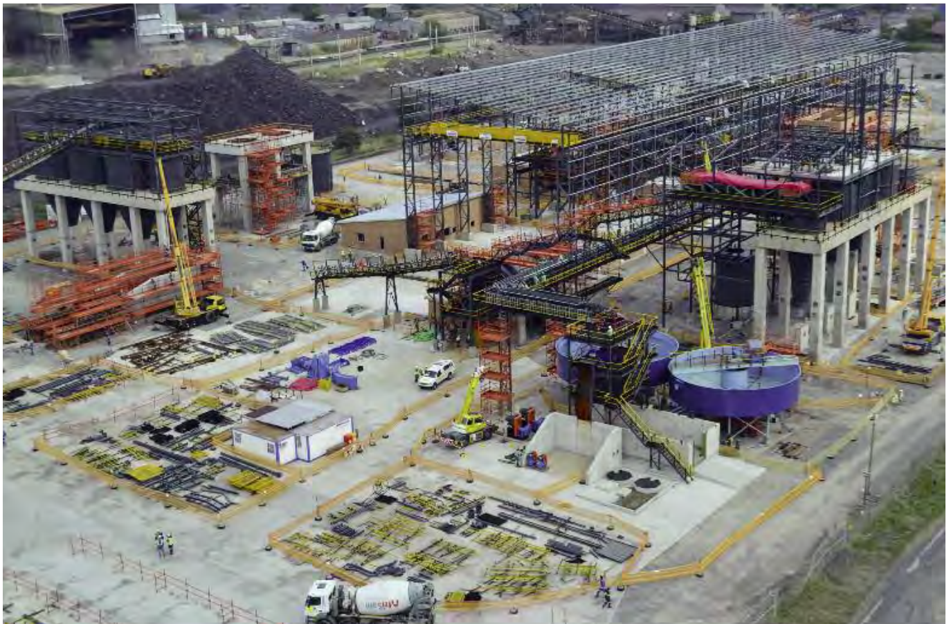
Sinter plant during construction.
