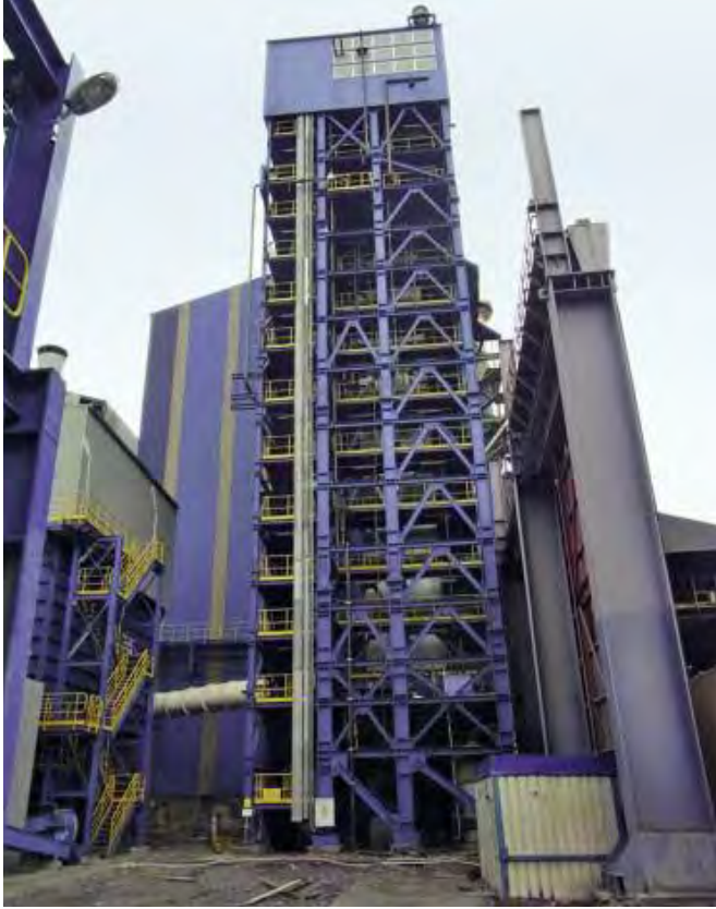
Energy recovery system erection.
