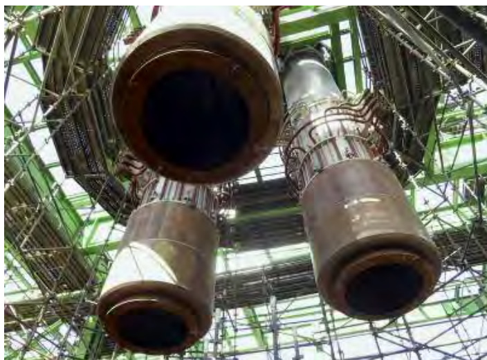
Installation of electrode at Lion.
