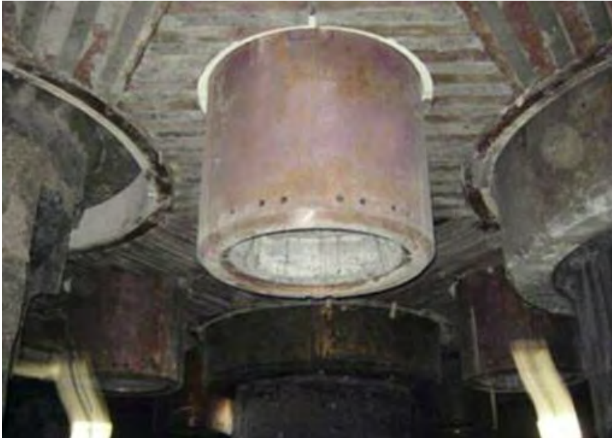
Water-cooled copper roof after several years of operation.
