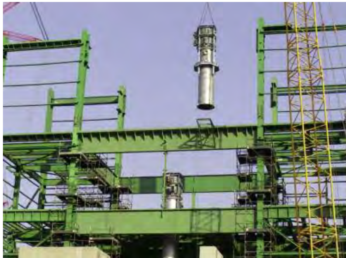
Installation of the equipment for Lion.
