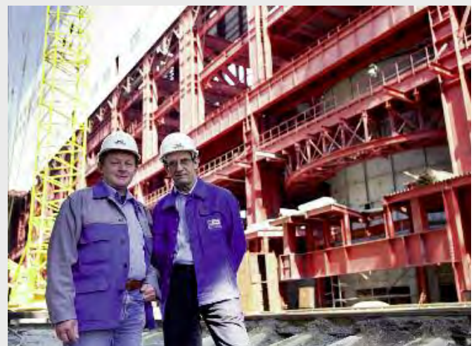
Kazchrome plant during construction.
