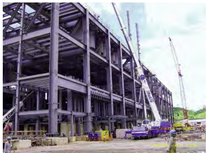
MOP plant during construction.
