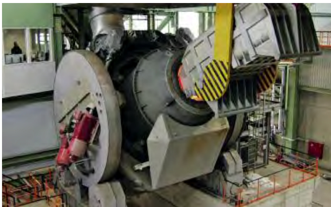
TBRC converter for copper production.
