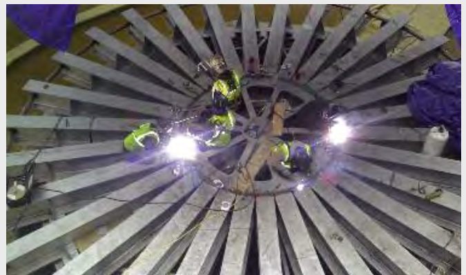
Welding grillage beams.
