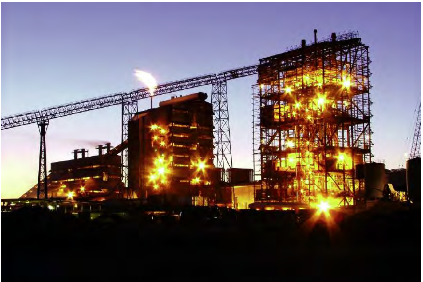
Heric plant at night.
