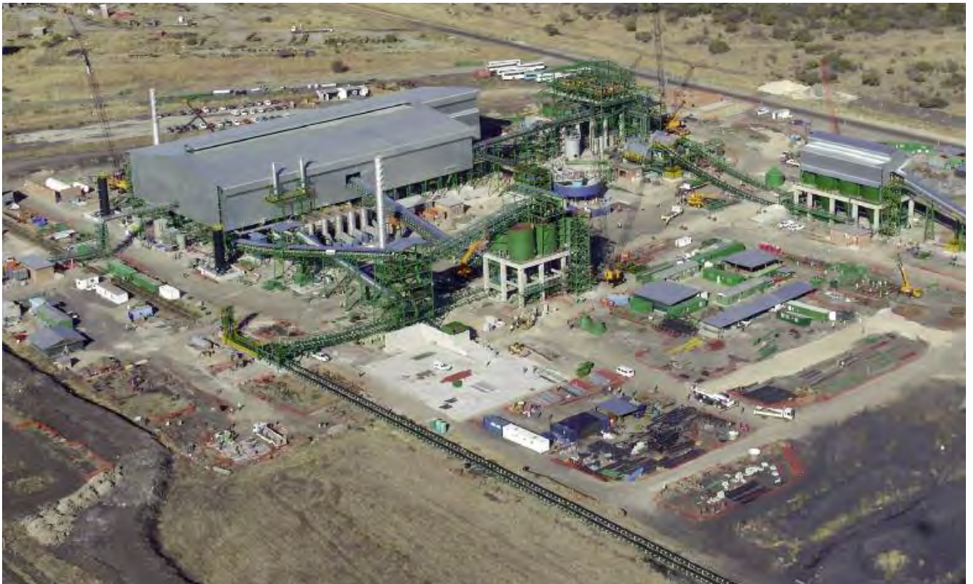
Sinter plant during construction.
