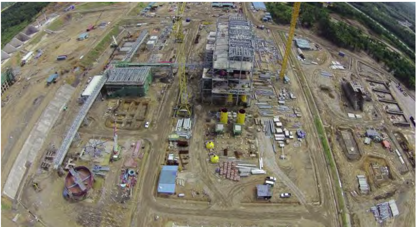
Sakura plant during erection.
