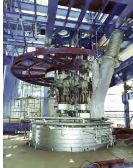
Construction of a smelter.
