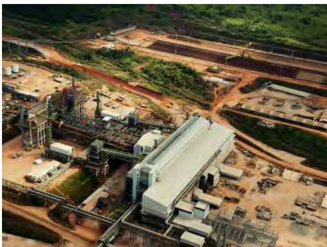
Top view of the MOP plant in Brazil.
