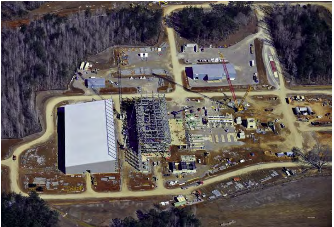
Mississippi Silicon plant during construction.
