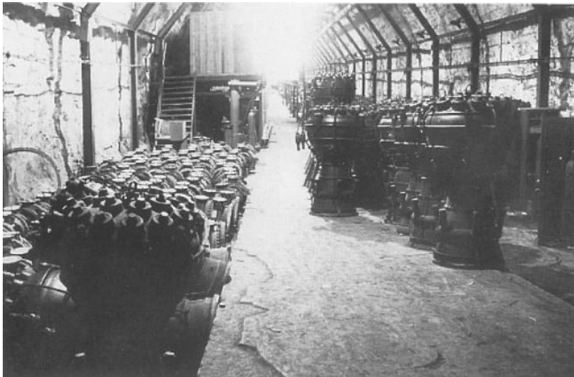
Combustion Chamber Storage
