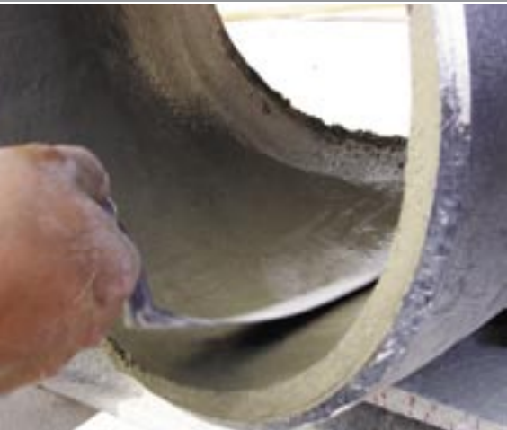
Hand applied cement mortar
