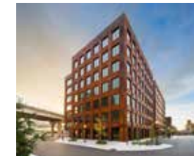
Project Type: Office Location: Minneapolis Award: Architizer A+ Awards Architect: Michael Green Architecture
