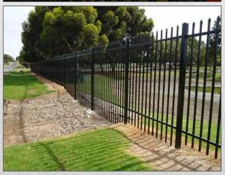
Palisade fencing is made-toorder, hot-dip galvanized or PVC coated steel. These fences are often over 4 meters high, topped with pales to deter climbers.
