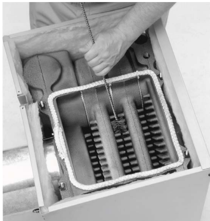
Cleaning Boiler Flueways Figure 3
