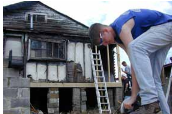
Habitat volunteers fix an old house in Birmingham, Alabama.
