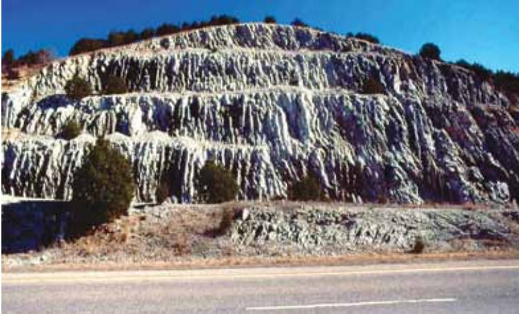
Figure 3. Viola Limestone along the I-35 roadcut. This is the deepest cut in the Arbuckle Mountains, with a vertical span of 156 feet, Murray County.
