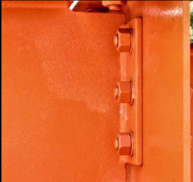
Shear End Plate Connection
