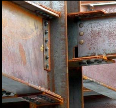
Bolted Flange Plate Connection
