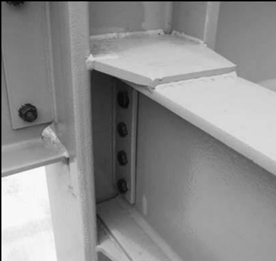
Welded Flange Plate Connection
