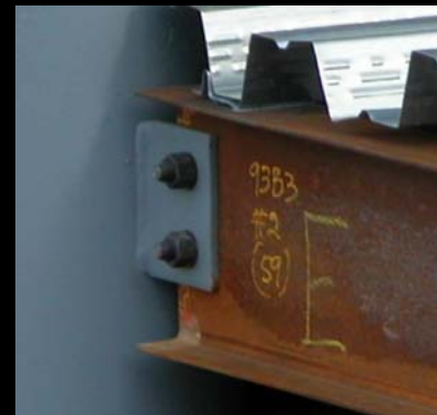
Single Plate Connection (Shear Tab)
