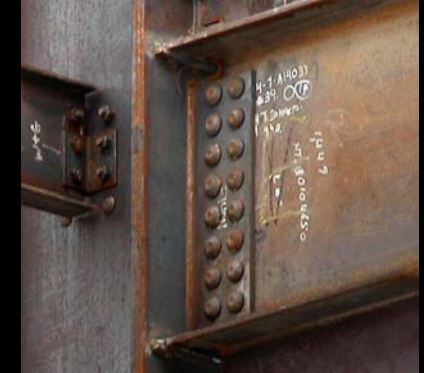
Welded Flange Connection
