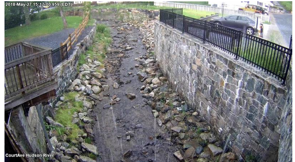
Court Avenue Culvert
