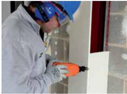
Where boards abut at corners Glasroc F FIRECASE boards are fixed together at 150mm centres with suitable length Glasroc F FIRECASE Screws.
