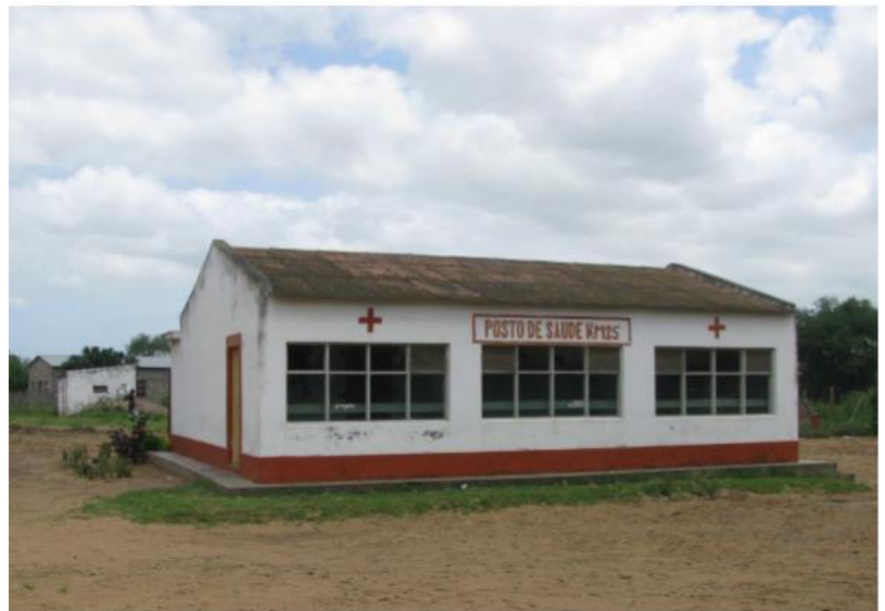
Figure 1: Rural area clinic that is also used as a warehouse
