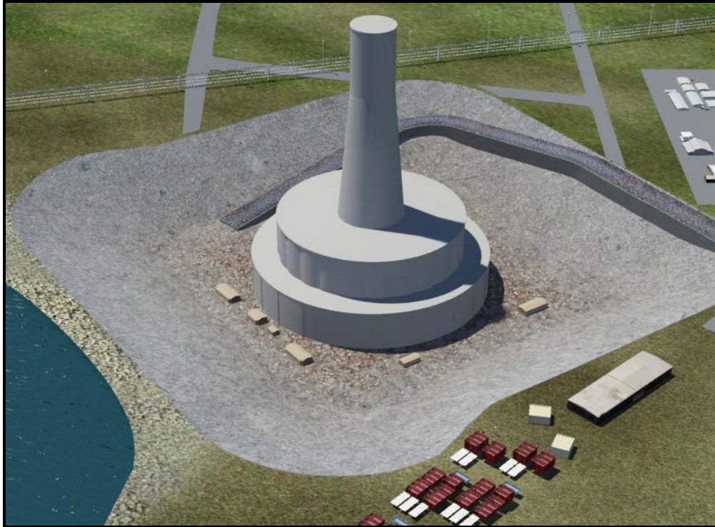
Figure 2-1 Proposed Concrete Gravity Structure
