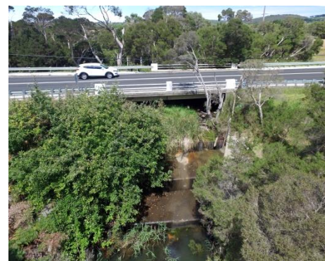
Littlejohn Bridge, over Dunn's Creek
