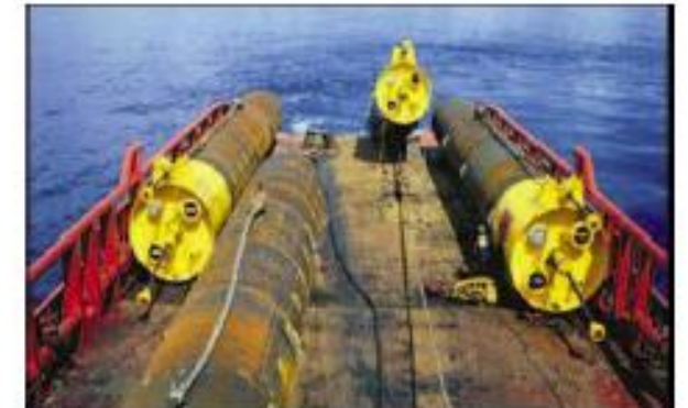
Figure 17 Multiple Suction Piles Installed from Single Vessel
