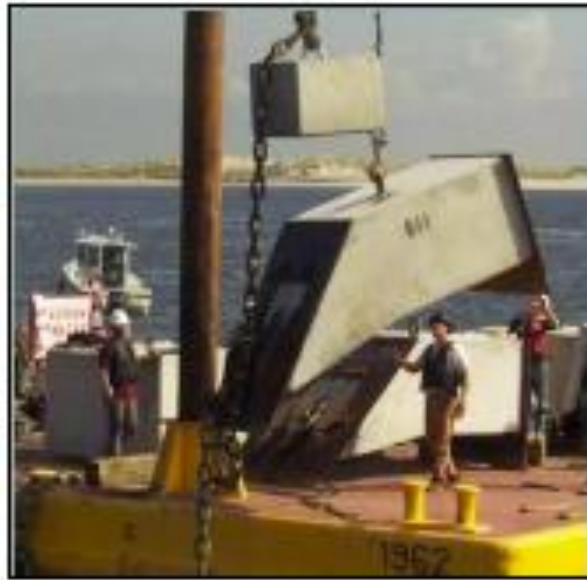
Figure 13 Enhanced Deadweight Anchor
