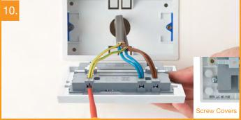
Make sure that the wires are fully inserted into the terminal and that no bare copper wire is visible. Tighten the screws securely onto the copper wire, not the outer sheeting. Before fixing remove screw covers from rear.
