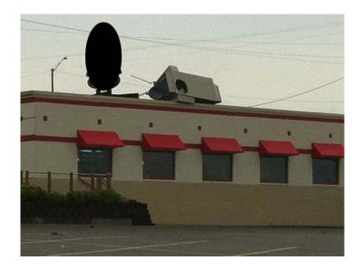
Overturned unit, exposing the building and its occupants to the wind and rain. Also, the gas lines have been bent and possibly damaged.
