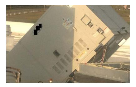
In 2012, Superstorm Sandy was another jarring example the importance of effective wind restraint of mechanical equipment. Due to the storm hitting such a largely populated area, the number of bad installations was significant. Many of these installations showed failure at the attachment to building structure.
