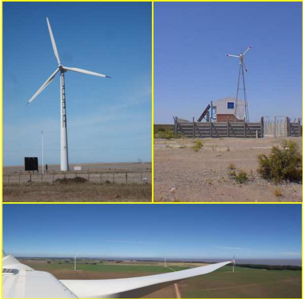
Fig. 9. Wind turbines (WT) of different powers, exhibiting aerodynamic different solutions; (top at the left side) WT of 600kW in the wind farm Bajo Hondo in Punta Alta, Argentina, with brake in tip of blade; (top at the right) small WT of 1kW for autonomous supply of relay station of micro waves in surroundings of Puerto Madryn, Argentina; (below) blade of WT of 2 MW in Magdalena's wind farm (Uruguay).
