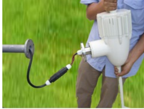
4、 LAY THE CABLE THROUGH THE TOWER
