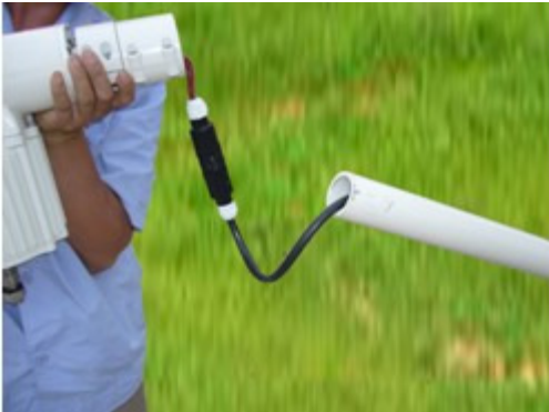
5、 LAY THE CABLE THROUGH THE TOWER
