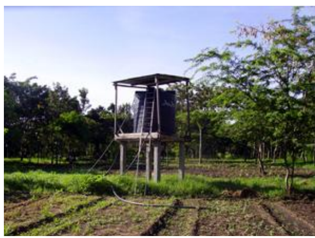
Figure 15. Water tank A at ATC.
