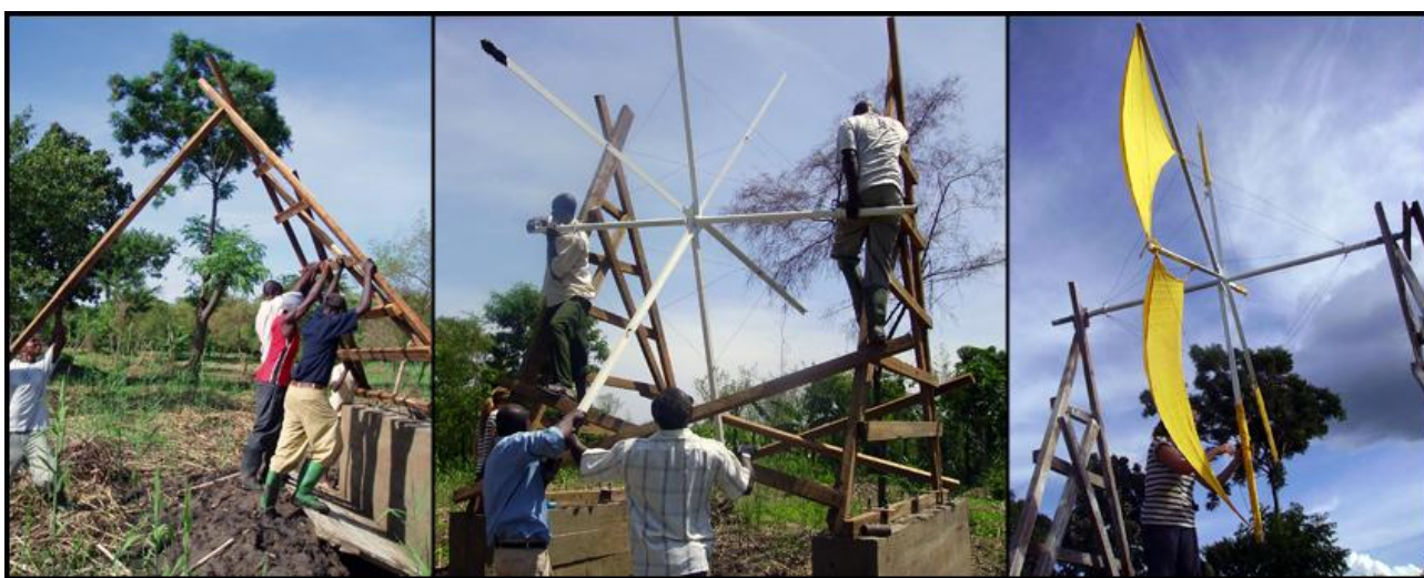
Figure 26. Putting the windmill together.
