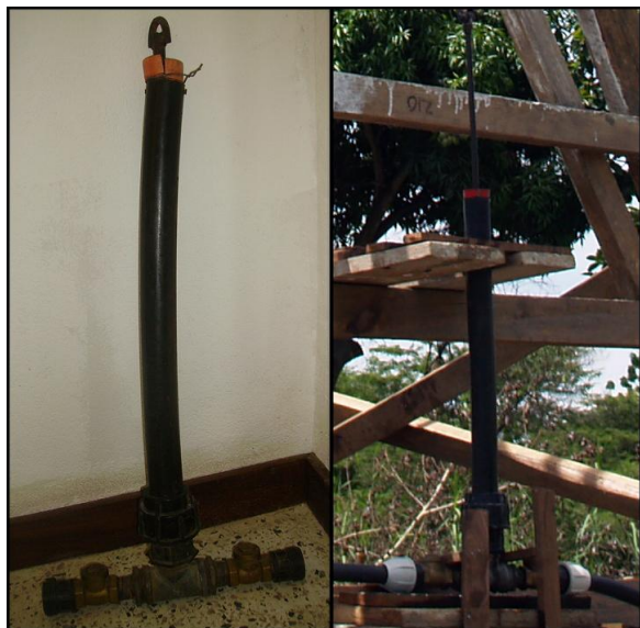
Figure 27. Pump before and after restoring.
