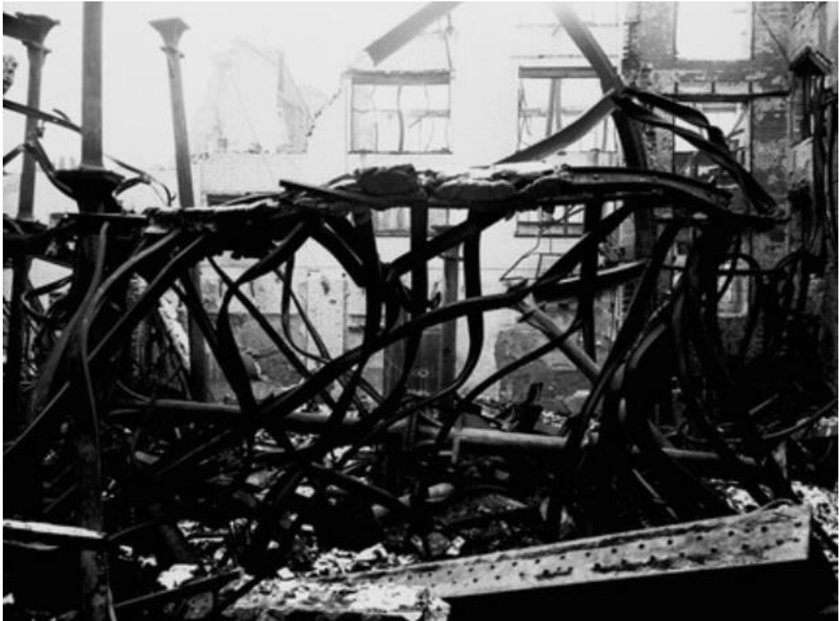
Bomb damage, Salisbury Square, EC4, December 1940
