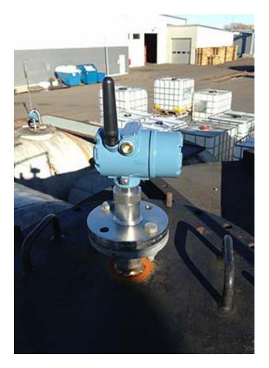
Figure 1. This wireless guided wave radar device is being used to measure tank level, an application particularly well suited for wireless as connecting a wired device would be difficult due to the hard to access location. (Courtesy of Emerson Process Management)
