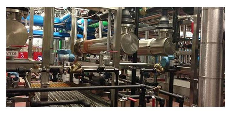
Figure 2. Wireless instruments can be used to monitor variables on equipment such as heat exchangers, pumps and piping systems. (Courtesy of Emerson Process Management)
