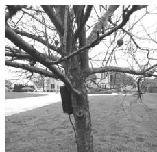
DA-611TO installation with the Sensor buried under the drive and the Transmitter hidden/mounted on a nearby tree.
