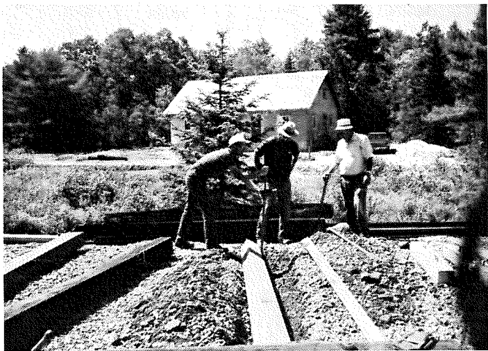
L to R: Jeff Schumaker, Bruce Wilson and John Bradbury setting 1 of 6 very heavy sills for Bay #3
