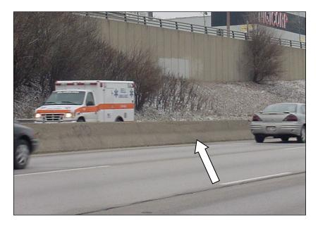
Figure 2.9.3.4-1: Concrete Median Barrier Wall.
