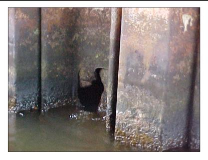
Figure 2.9.4.1-1: Cell Dolphin Deterioration.
