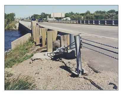
Figure 2.9.5.1-1: Cable Guard Next to a Beam Guard.
