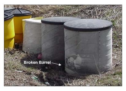
Figure 2.9.5.3-1: Damaged Impact Attenuator.
