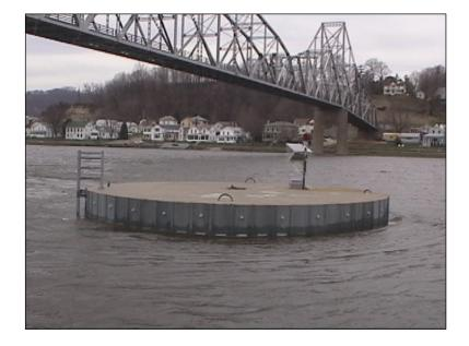
Figure 2.9.2.1-1: Cell Dolphin During Flood Conditions.
