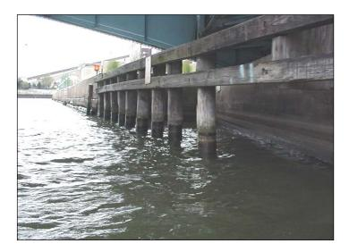
Figure 2.9.2.3-1: Independently Supported Timber Fender System.
