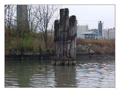
Figure 2.9.4.2-1: Pile Cluster Dolphin Deterioration.
