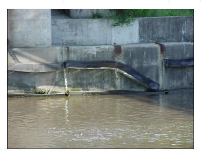
Figure 2.9.4.3-1: Failed Rubber Fender System.
