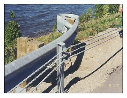
Figure 2.9.3.1-1: Section of Cable Guard Next to a Steel Plate Beam Guard.
