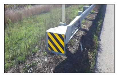
Figure 2.9.3.2-1: Newly Installed Beam Guard.
