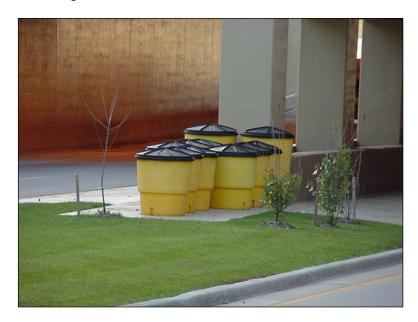
Figure 2.9.3.3-1: Impact Attenuator System.
