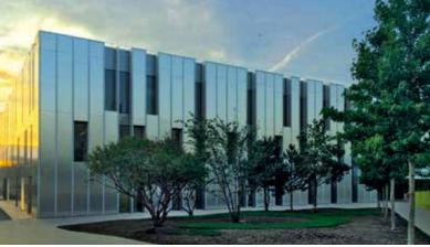
Pre-fabrication of elements in the factory has remarkably speeded assembly works thus allowing the installation of up to 600 m² of roof elements per day. In addition, this lead to a considerable reduction of on-site waste. Expensive disposal costs could be avoided and excess materials were recycled. Despite adverse weather conditions, works were concluded according to schedule.
