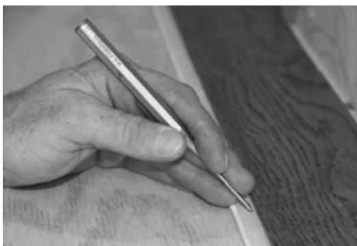
Fig. 6 Nail is completely lowered
