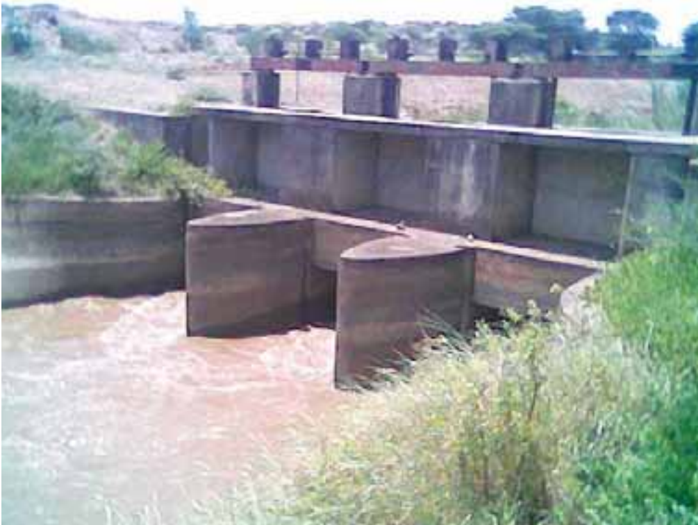
Figure 16. A concrete intake at Metahara near Awash River.
