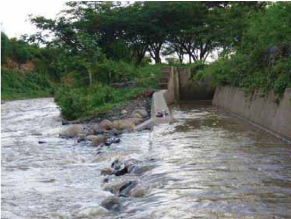
Figure 37. Modern diversion structure constructed by LWF at Kolla Shara.
