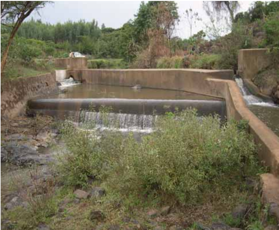
Figure 49. Indris Weir supplies irrigation water to five WUAs.
