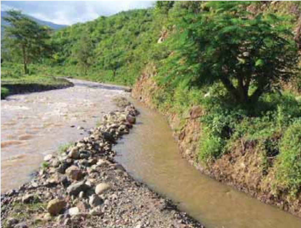
Figure 38. Traditional diversion structure at Chano Dorga.
