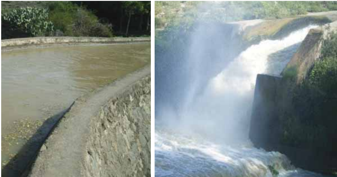
Figure 17. Canals made of stone masonry and inclined plane are used to supply irrigation water to the field.
