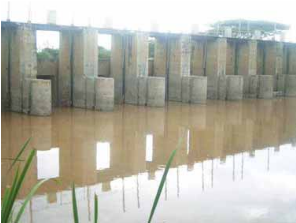
Figure 61. A barrage with nine bays is used to divert irrigation water for Bilate Irrigation Scheme.
