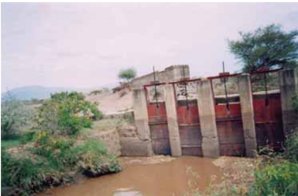
Figure 31. The main intake structure with manually operated gates at Nura Era.
