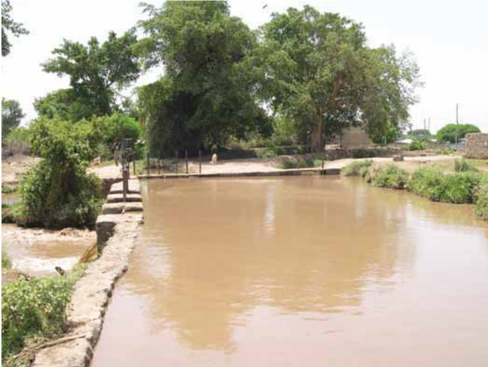
Figure 57. A silting basin is employed to reduce the sediment load of water from the Awash River for irrigation.
