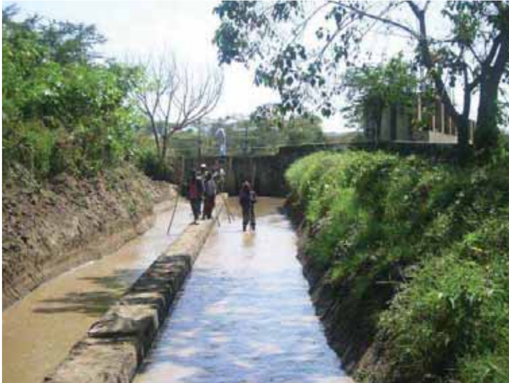
Figure 62. Main canal of Bilate Irrigation Scheme.
