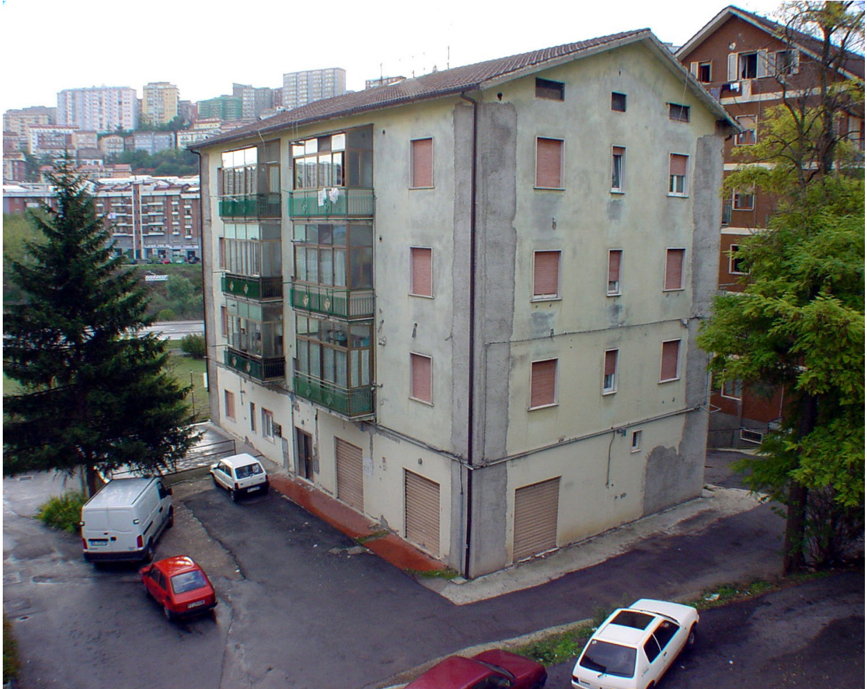
FIGURE 1B: Typical Building
