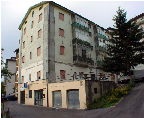
FIGURE 1A: Typical Building
