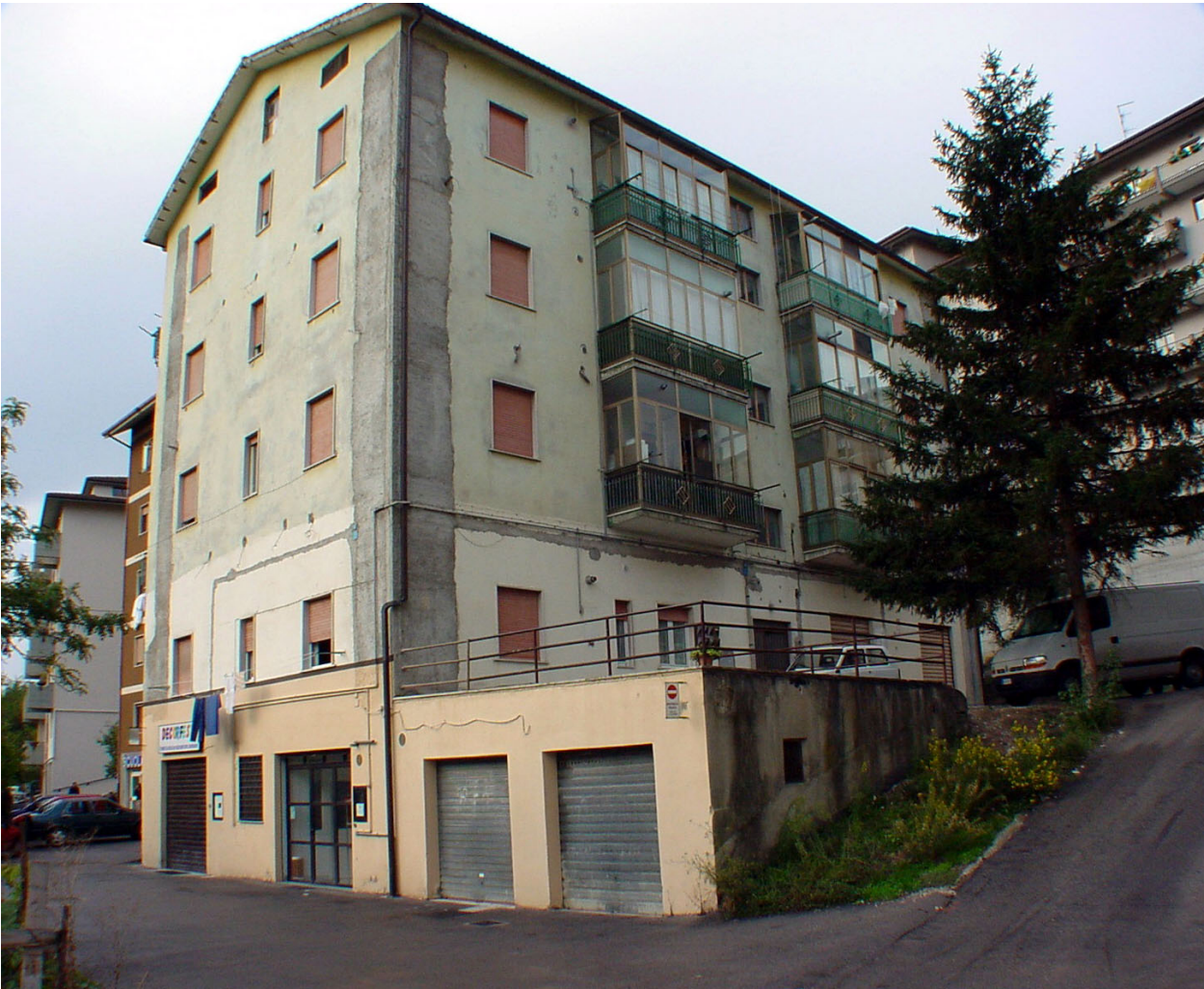
FIGURE 1A: Typical Building
