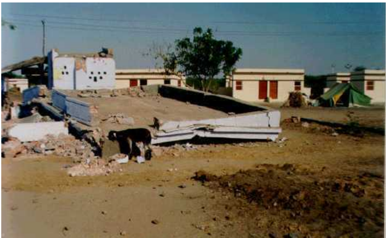
FIGURE 6J: View of a collapsed traditional brick masonry building in cement mortar (foreground) and masonry building with lintel bands which sustained only a moderate damage in the 2001 Bhuj earthquake (Source: IIT Powai, 2001)
