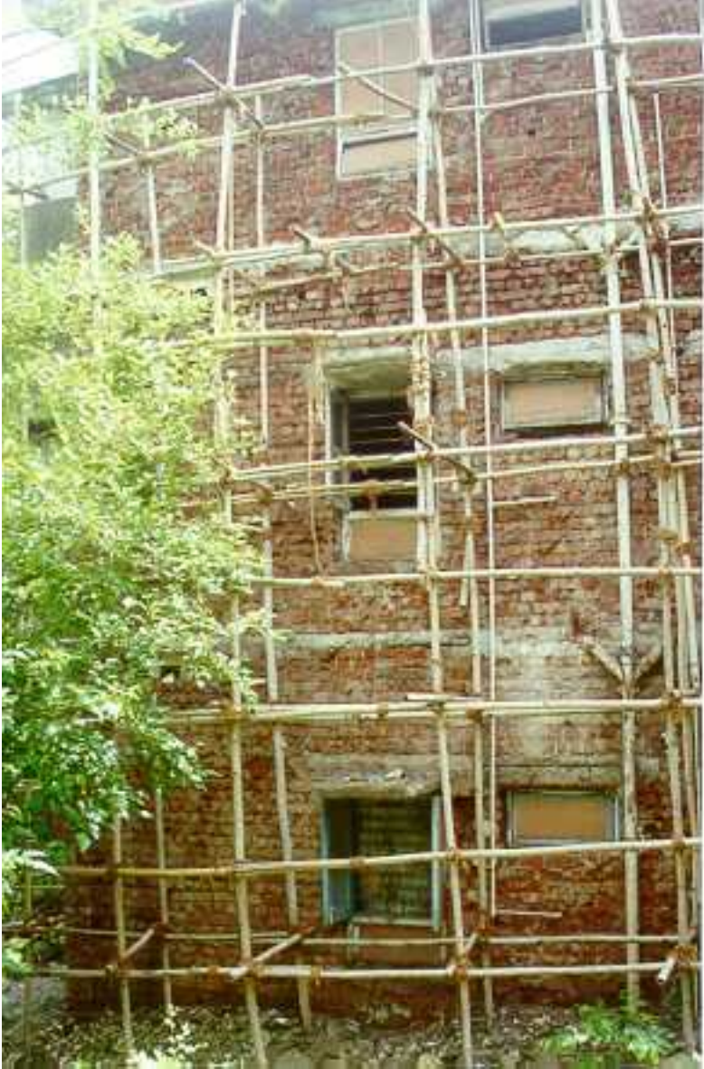
FIGURE 2A: Key Load-Bearing Elements - A Building Under Construction
