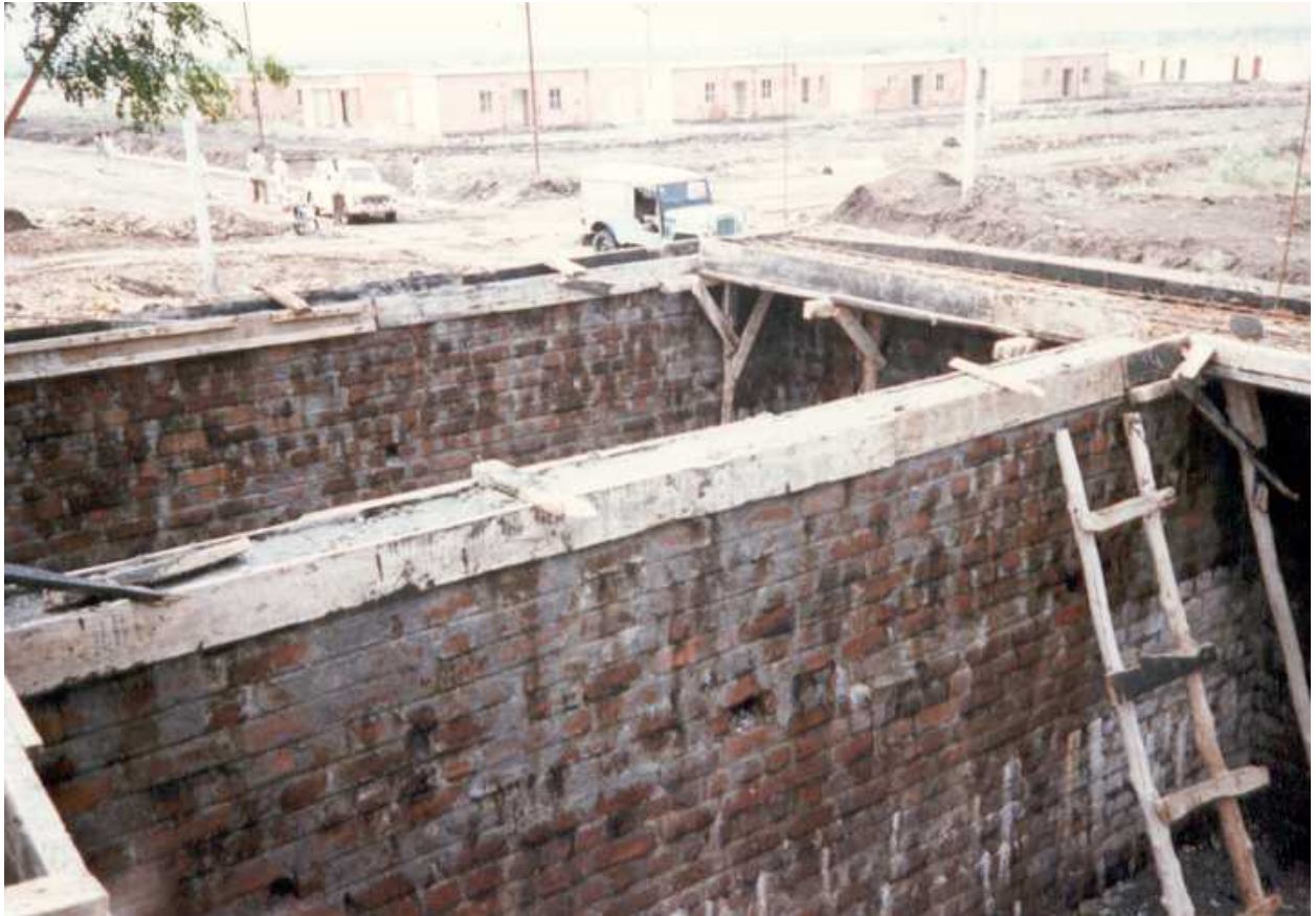
FIGURE 7F: Construction of RC Lintel Band - Pouring of Concrete Completed
