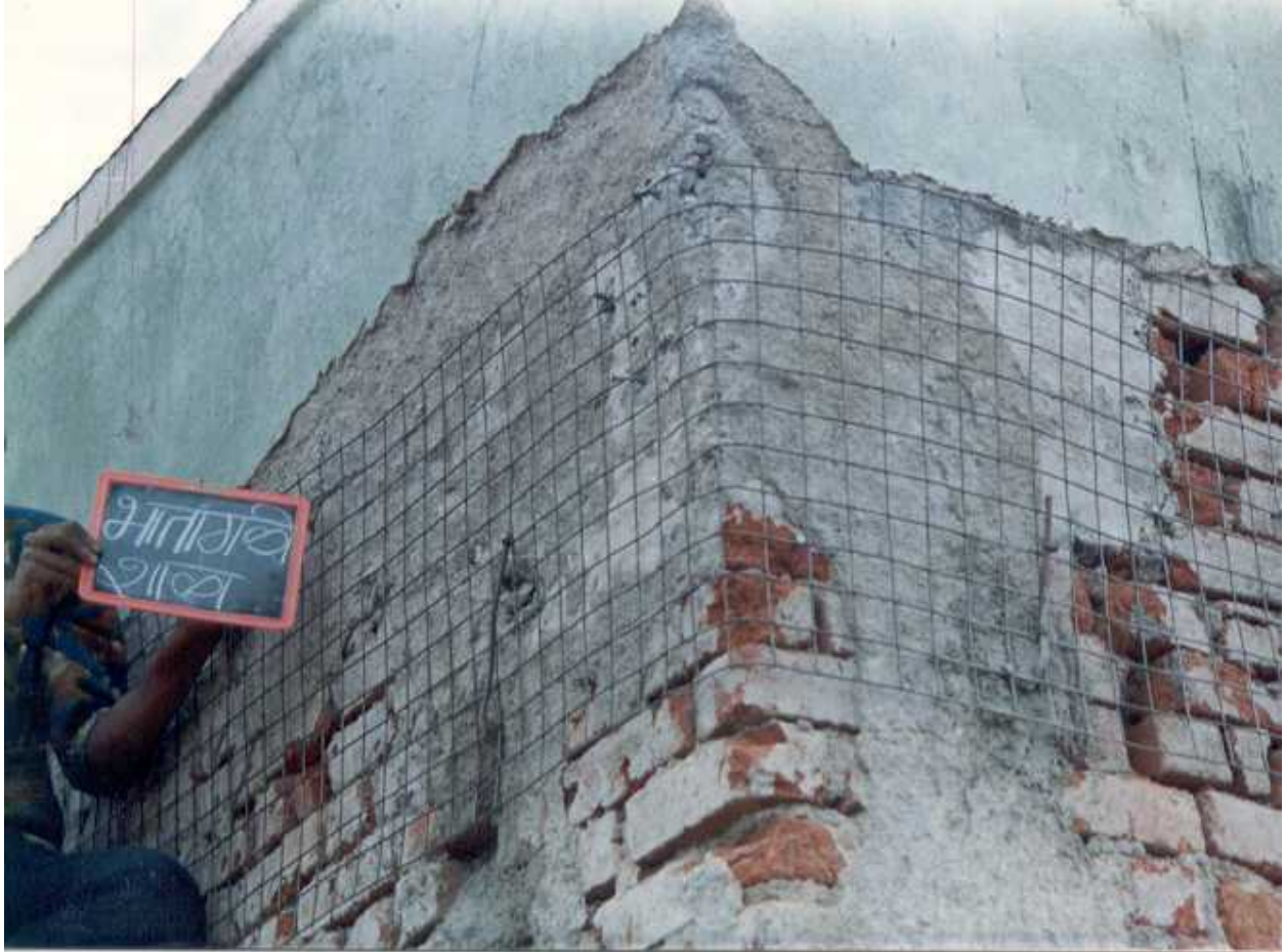
FIGURE 7B: Seismic Strengthening Techniques - Lintel Bandage
