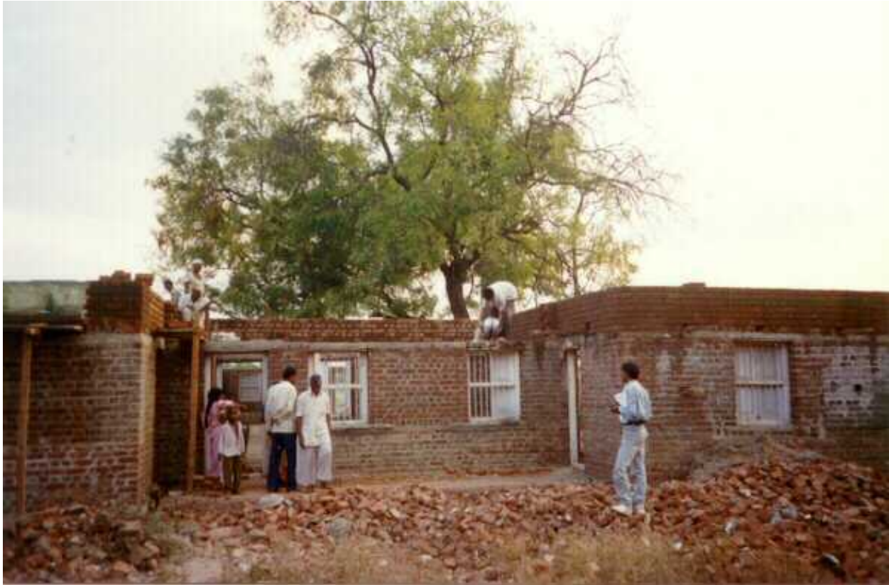
FIGURE 2B: Key Load-Bearing Elements - A Building Under Construction
