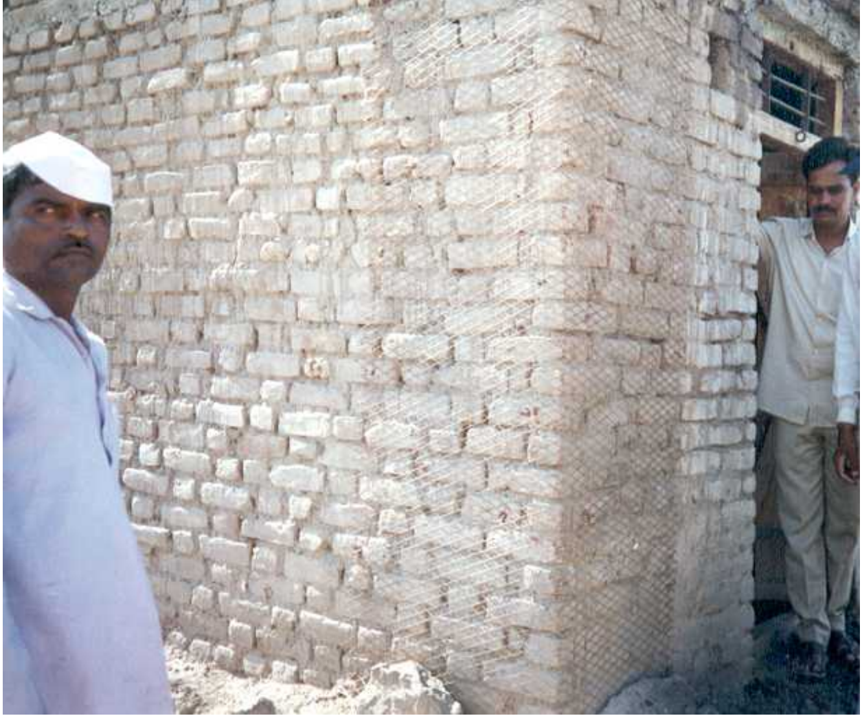
FIGURE 7C: Seismic Strengthening Techniques - Corner Strengthening
