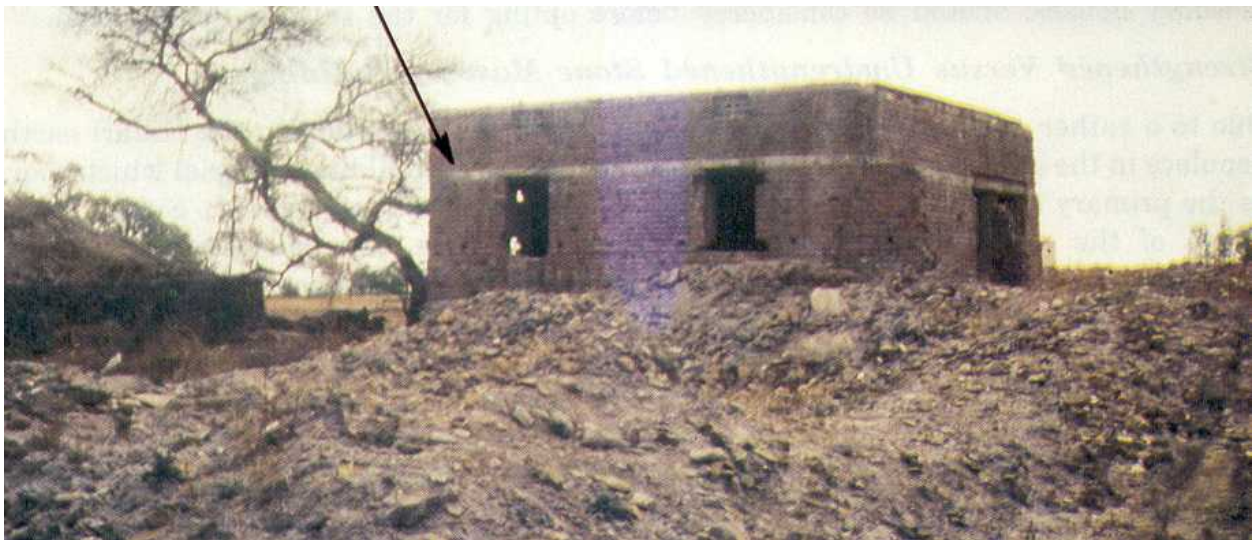
Figure 5A: Key Seismic Resilient Features - RC Lintel Band and Good Quality Construction; note example of a building that sustained the effects of the 1993 Killari earthquake (M6.4) without damage, although located very close to the epicentre
