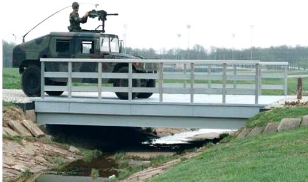
Figure 1. Vehicular bridge at Fort Leonard Wood, Missouri built in 1998 with a maximum load capacity of 12.5 tons.
