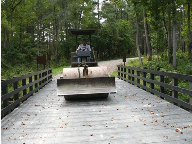
Figure 3. A successful crossing of a 30-ton steamroller over Bridge T85-19 at Fort Bragg, North Carolina.
