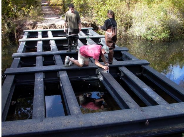
Figure 6. I-beam substructure of the Wharton State Forest bridge in New Jersey.
