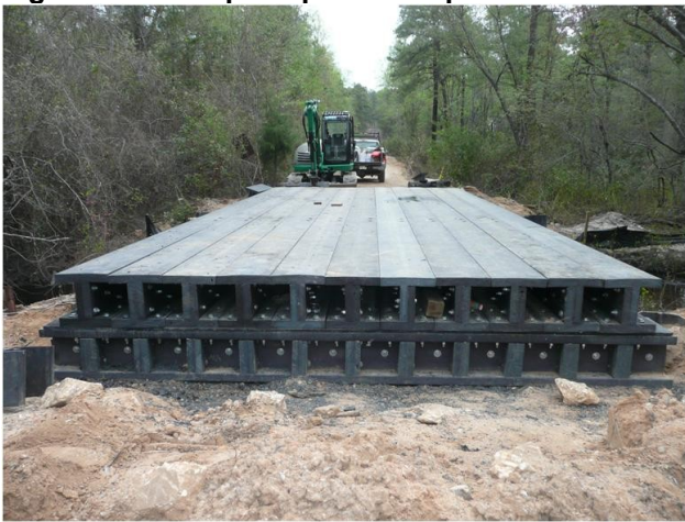
Figure 8. Girders installed on T85-18 spanning the length of the bridge.
