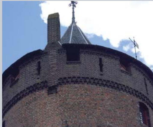
ABOVE Arrow slit with gun port, Muider Castle, the Netherlands. This castle dates to 1370 but was modified numerous times, so it is unclear when gun ports were added to all the arrow slits. (Sean McLachlan)
