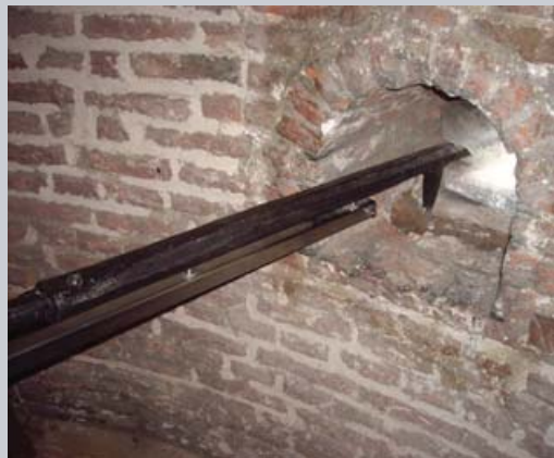
ABOVE A 15th-century hackbut positioned for firing at a gun port at Muider Castle, the Netherlands. Note the wooden crossbeam, now somewhat decayed, on which the hackbut could be braced. (Sean McLachlan)
