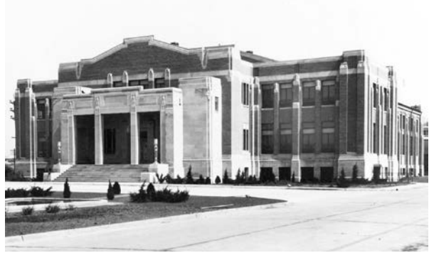
Building 12, Technical Data Library and Museum
