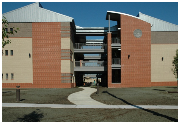
New Airmen's dormitory
