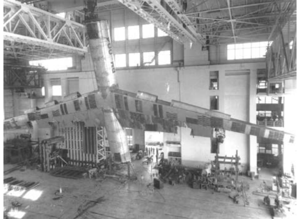
XB-36 fuselage and wing being prepared for structural testing in Building 65
