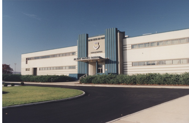
Building 262 became Headquarters Air Force Logistics Command in 1961
