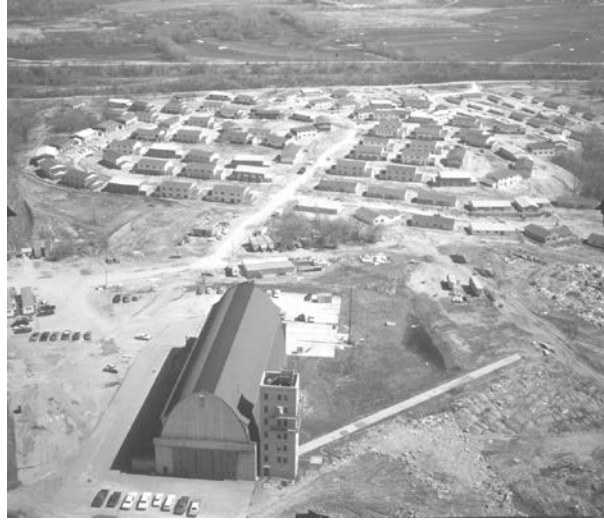
Woodland Hills housing complex under construction
