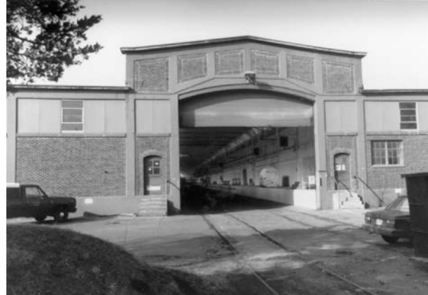
Building 1 with its covered trainway is the oldest military building at Wright-Patterson AFB
