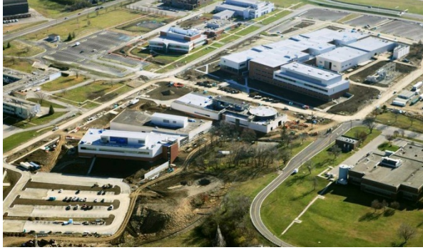
Construction on the Area B hilltop to house incoming BRAC units
