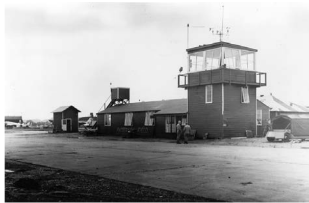
Patterson Field control tower, 1940
