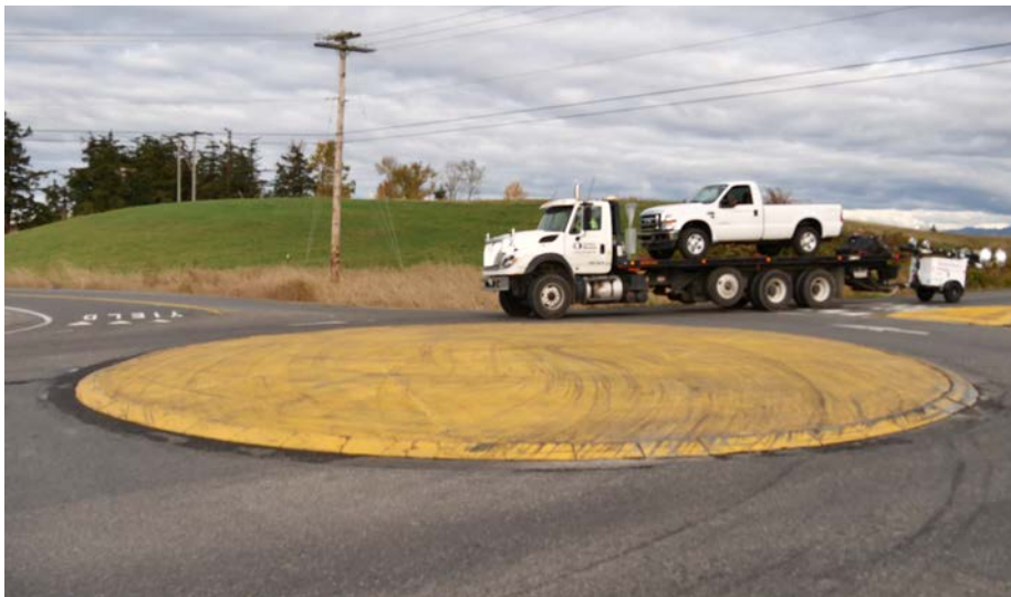
A truck navigates a compact roundabout. The truck apron (yellow, center) allows larger vehicles to drive over it because the turning radius in a compact roundabout is smaller than in traditional-sized roundabouts.
