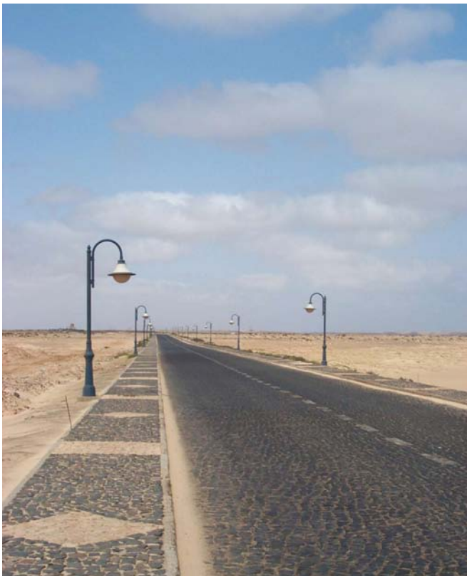
Infrastructure development. Sal, Cape Verde © WWF Germany / Birgit WEERTS
