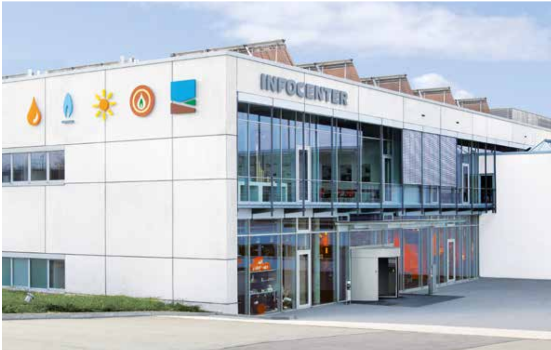
The Energy Centre and the Viessmann Academy in Allendorf
