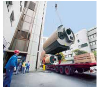
Delivery of a Vitomax boiler to site
