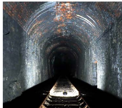
View of lined section of tunnel
