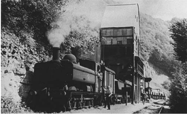
Tintern Quarry stone loading, September 1959
