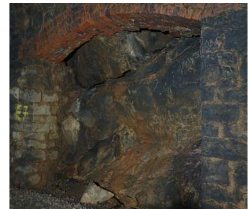
Alcove in tunnel wall
