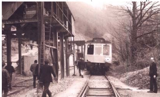
3: Quarry loading gantry next to railway
