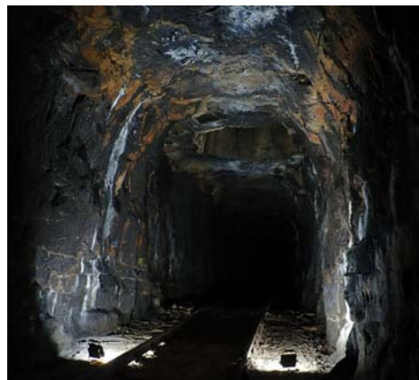
View of unlined section of tunnel
