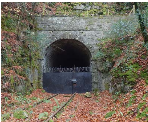
Northern portal of Tunnel
