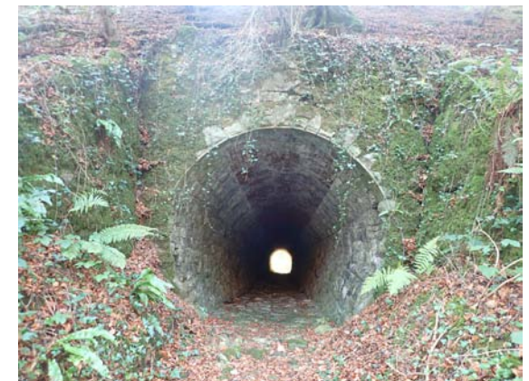
View looking through 60m subway
