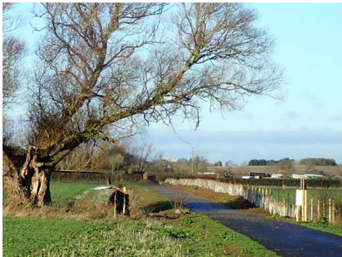
Waddesdon Greenway: constructed by Greenways, 2018
