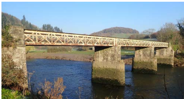
Wireworks Bridge – 3 spans, 200ft in length and owned by the Council
