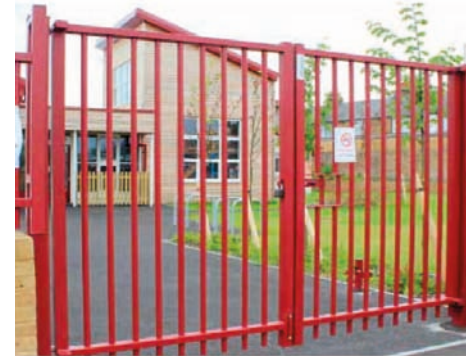
View of typical gates to be set 15m in from the portal so as to minimise disturbance to the visual aspect of the tunnel portals
