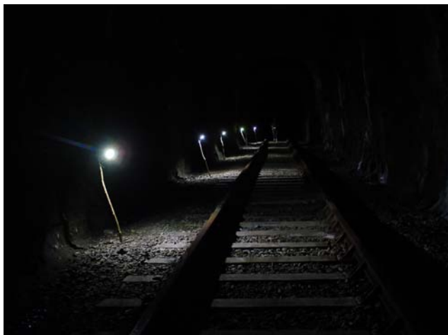
Picture showing lighting test in Tidenham Tunnel
