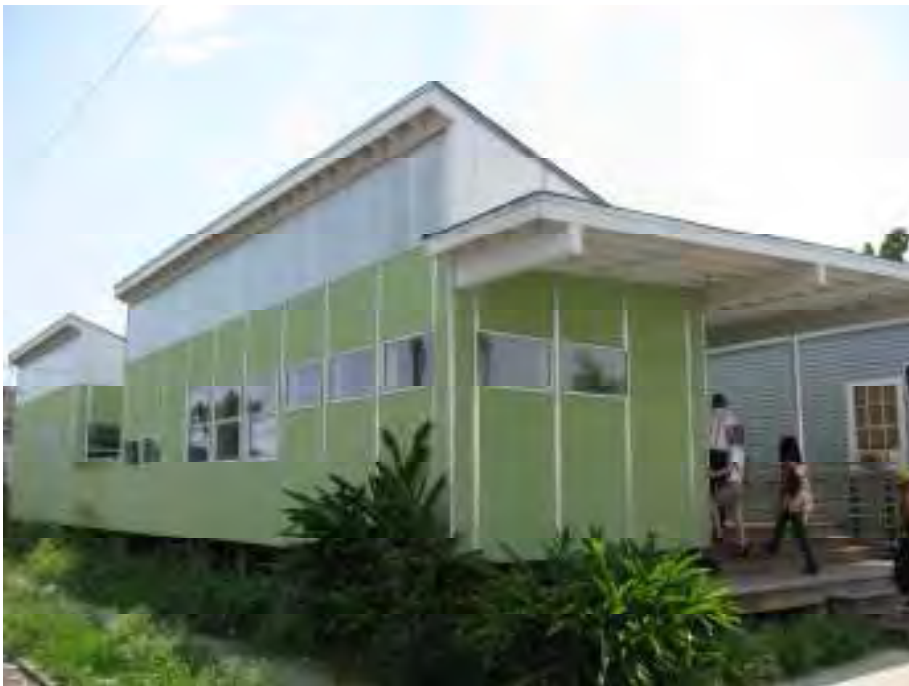
Tulane University's Tulane in Central City Greenbuild 1
