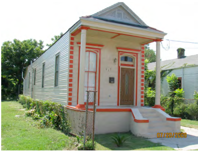
Figure 1. Shotgun house. This is a classic example of a vernacular New Orleans shotgun house: long and narrow with a generous porch and long overhang.
