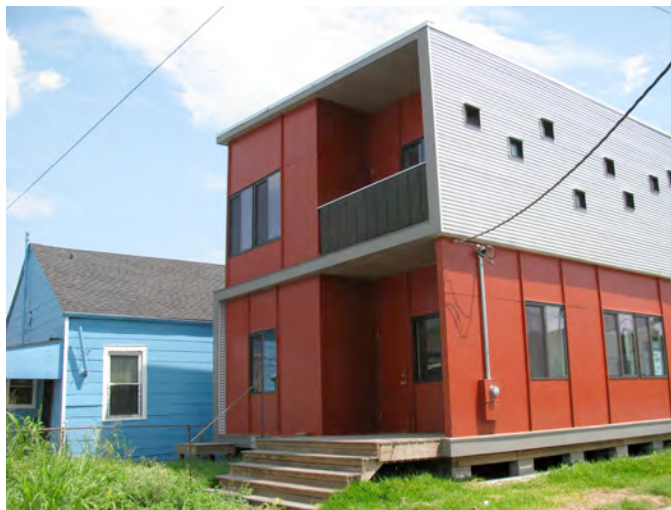
Figure 3. Tulane University URBANbuild Prototype 03. This house looms over the neighboring house.
