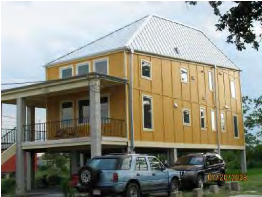
Make It Right house designed by Concordia Architects in Lower 9 th Ward (Type 4)
