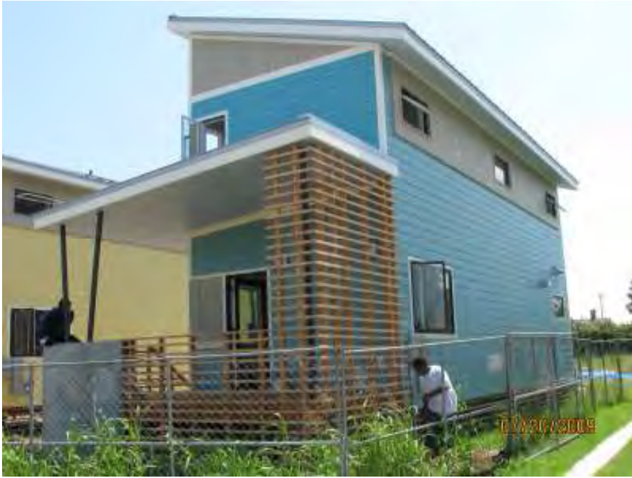
Global Green house in the Holy Cross District
