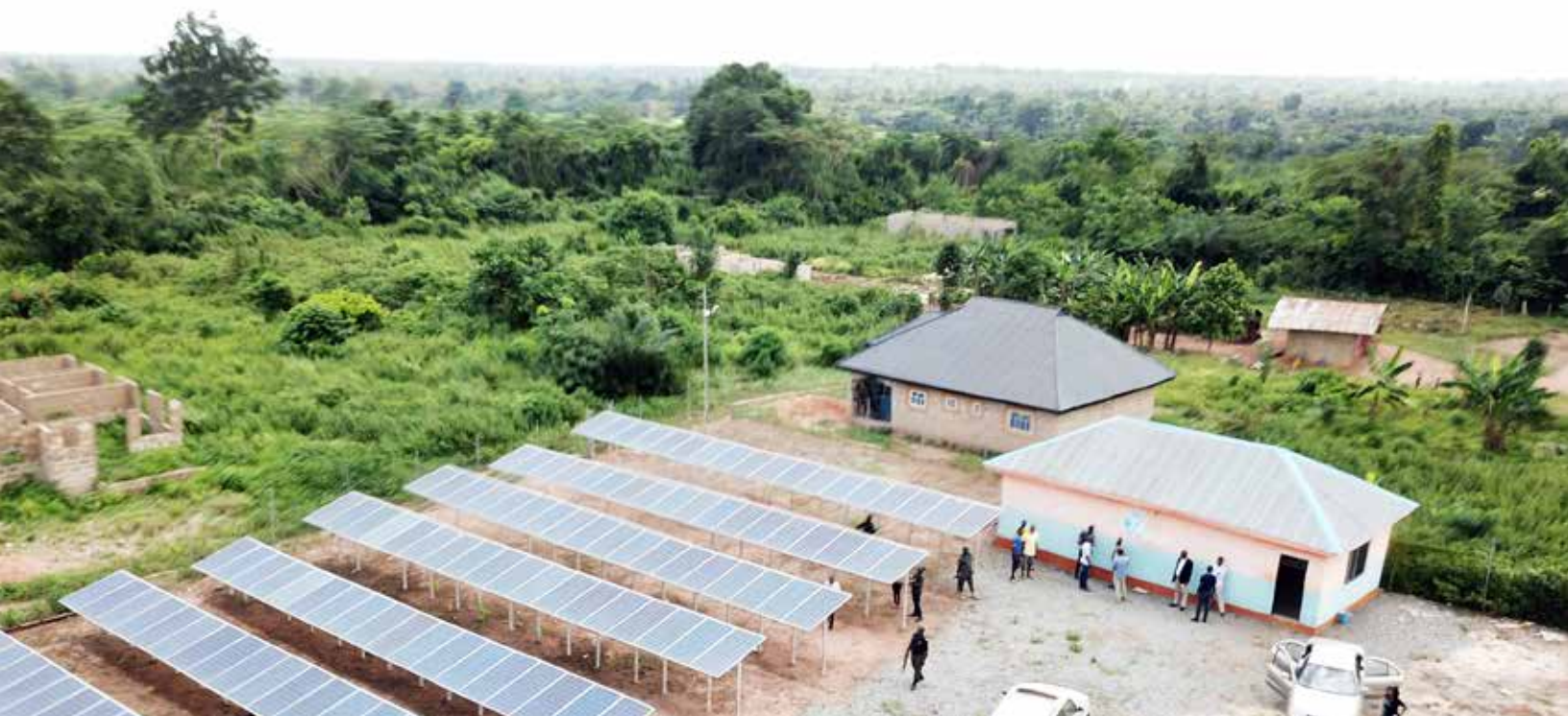
PHOTO: RMI SITE VISIT
